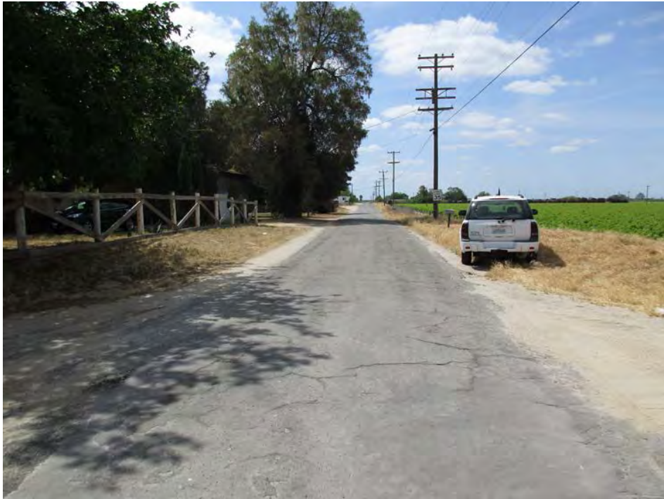
Hughes Avenue looking South
