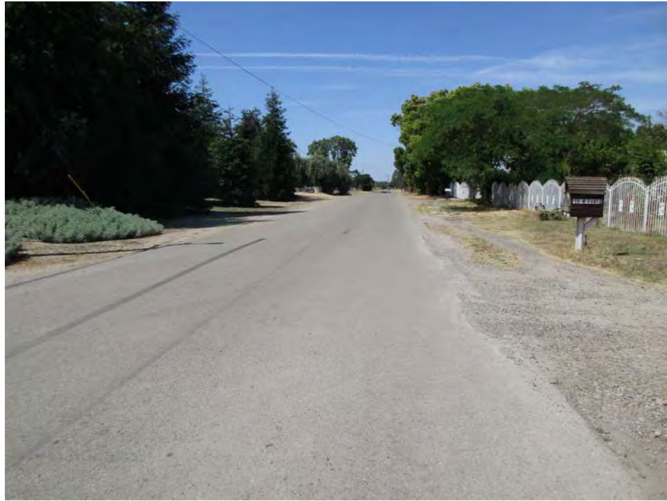
Typical Un-serviced Road looking North
