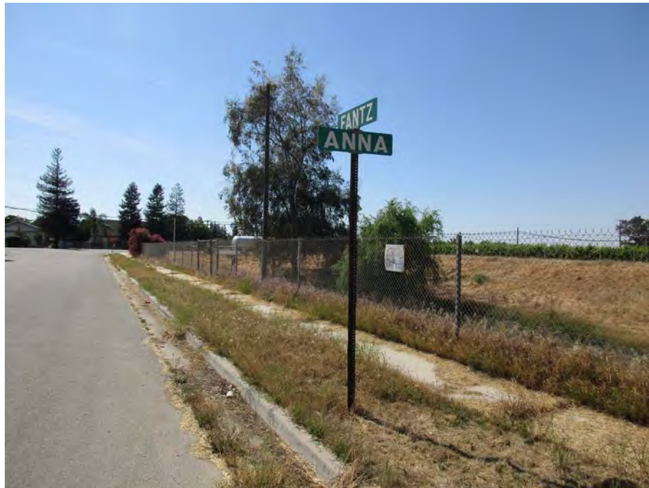
Stormwater Basin for Tract 1826 looking West
