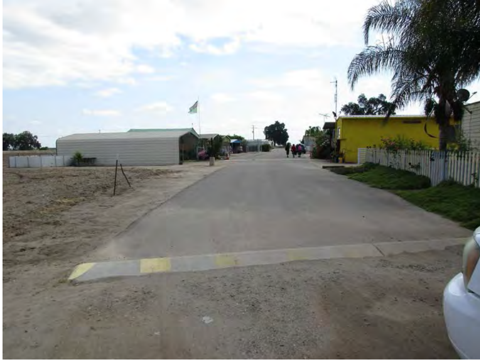
Northerly Road looking East
