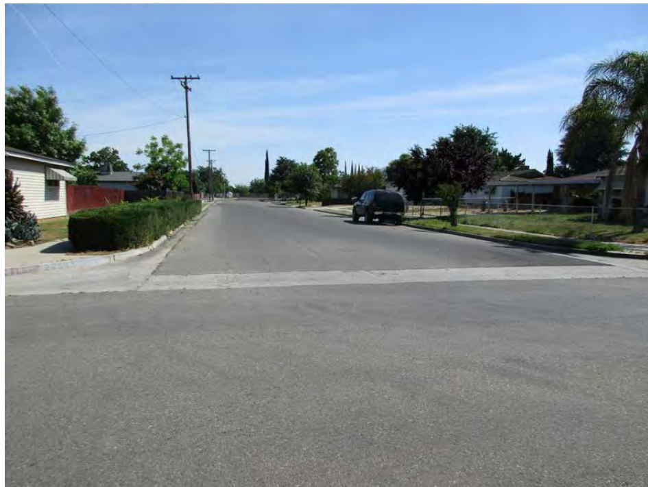
Typical Valley Gutter looking South
