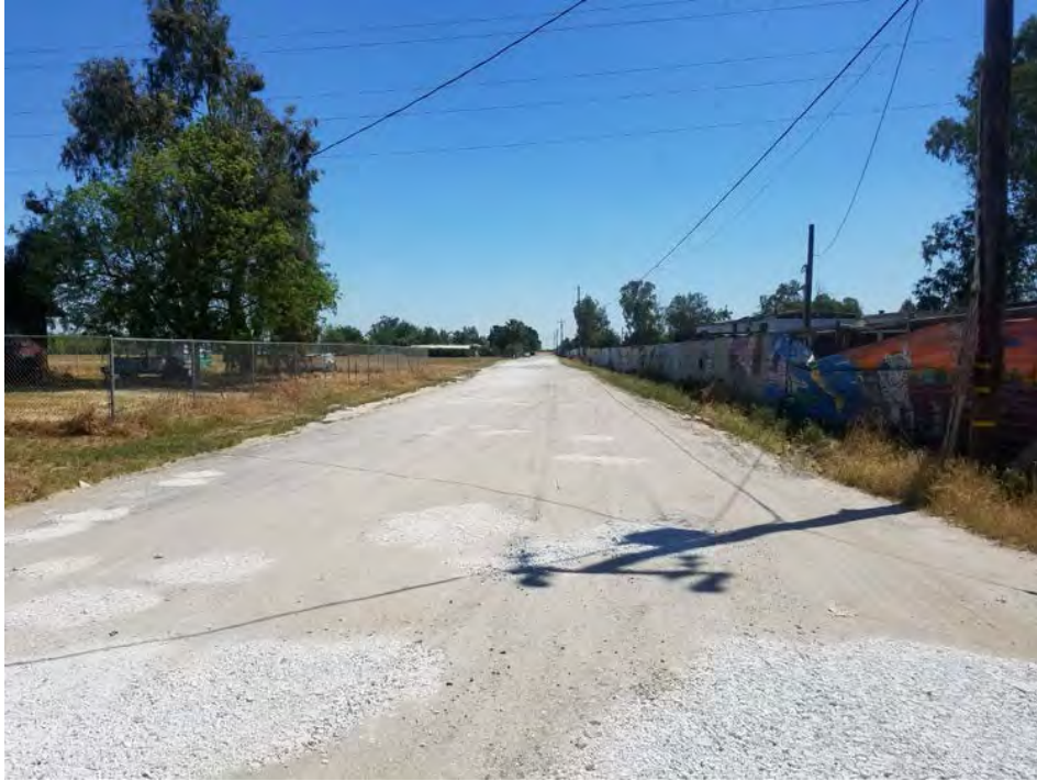
Northerly Road looking East
