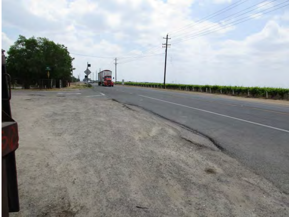
Madera Avenue looking South
