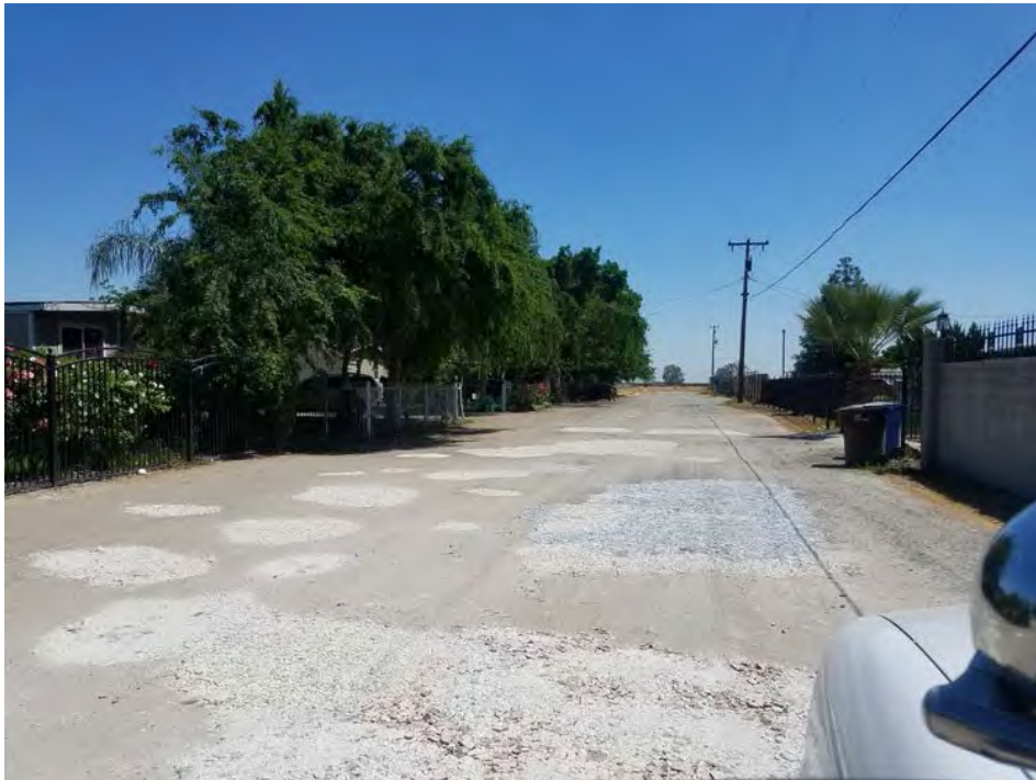
Northerly Road looking East
