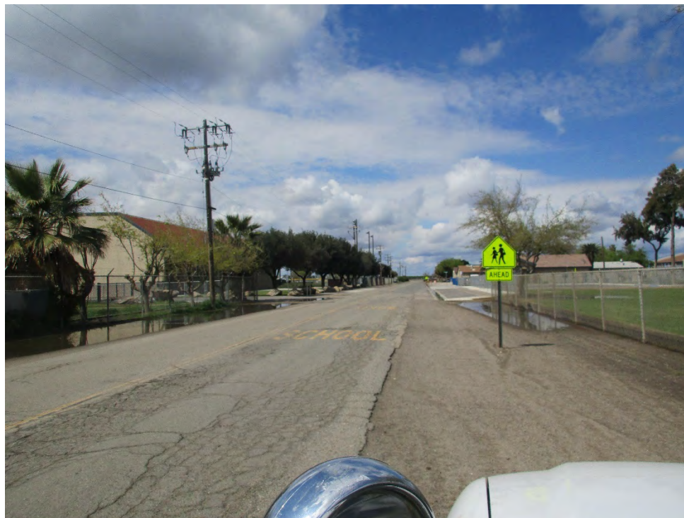
Randolph Avenue Looking Northwest – March 23, 2020
