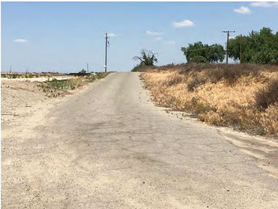
Looking North down Topeka from Avenell
