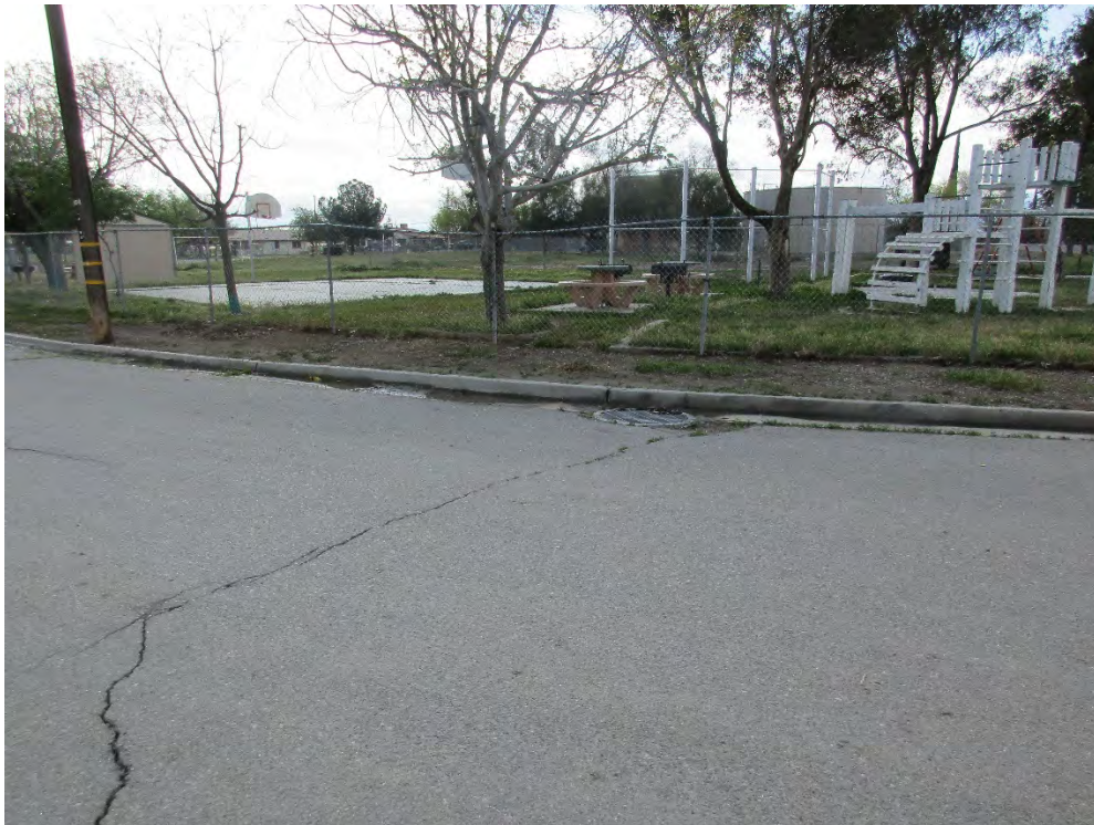
El Progreso near intersection with Hildalgo Avenue – March 26, 2020
