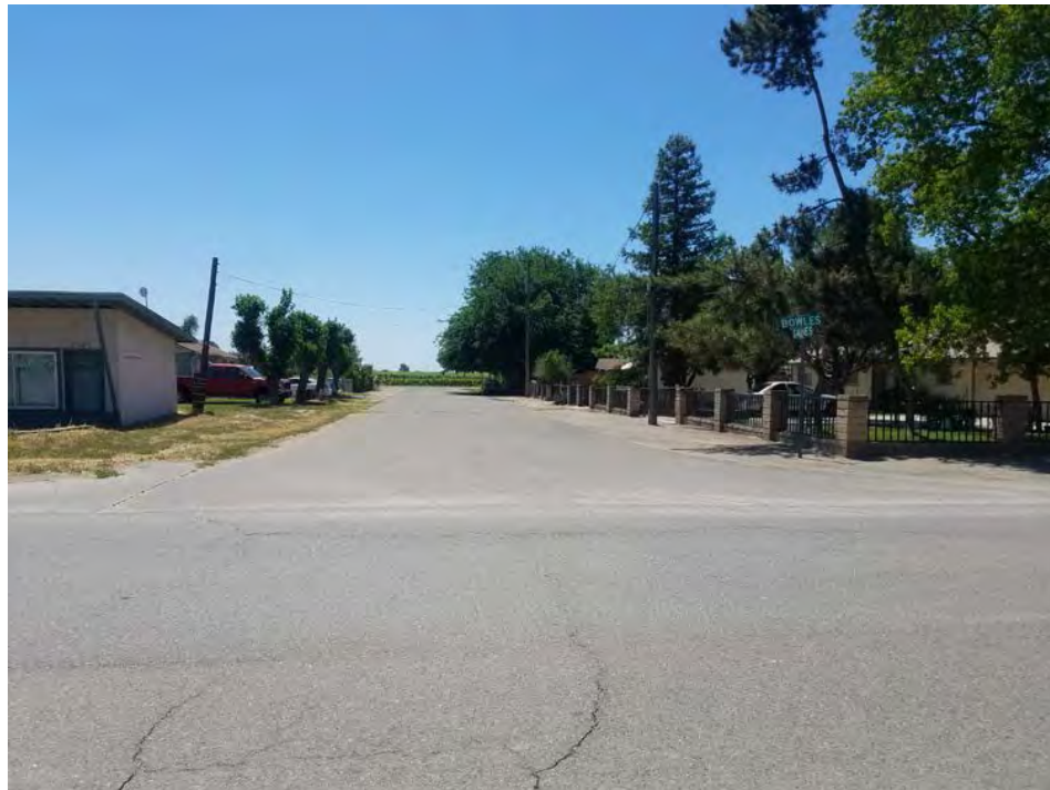
Gains Avenue looking South
