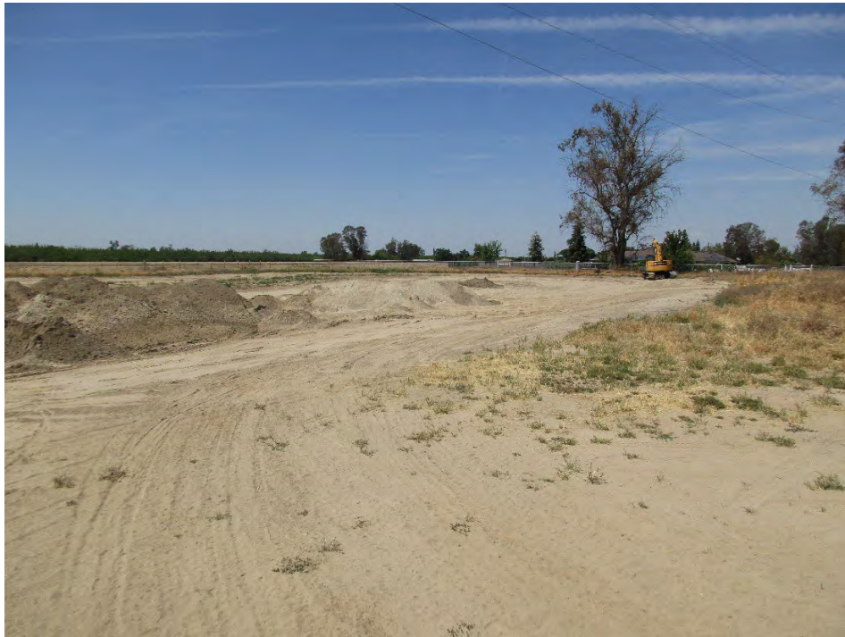
Primary Basin looking Northwest
