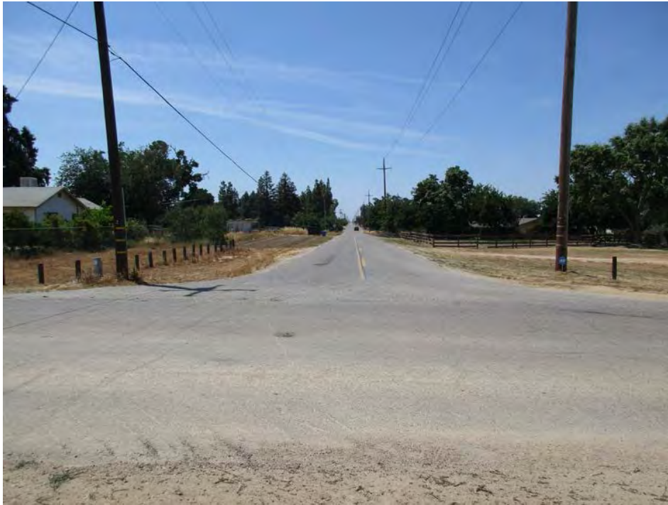
Ashlan Avenue looking West
