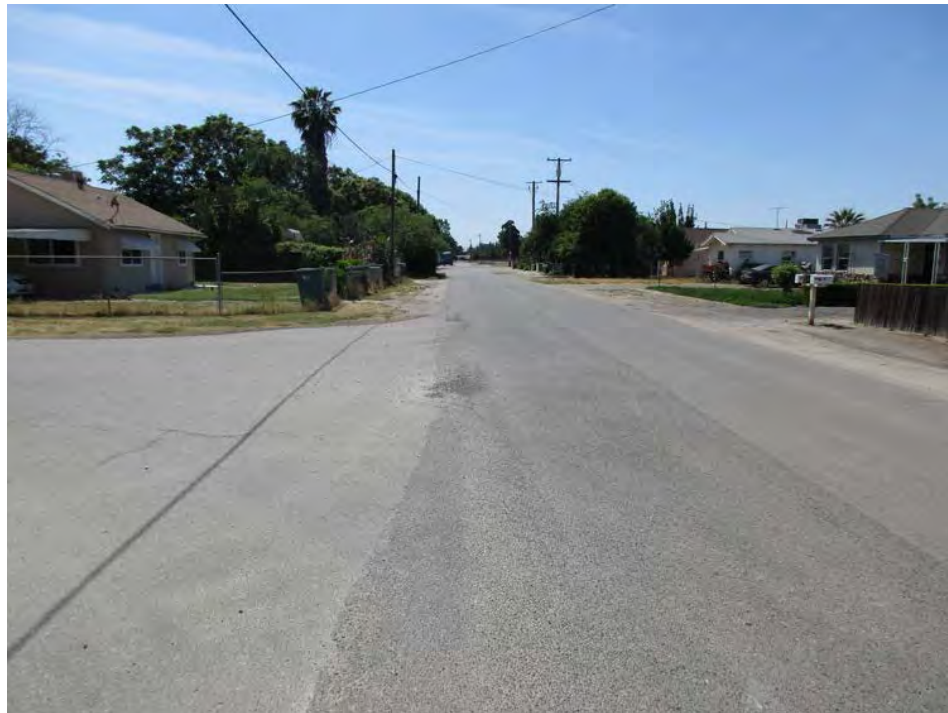
Typical Un-serviced road looking West
