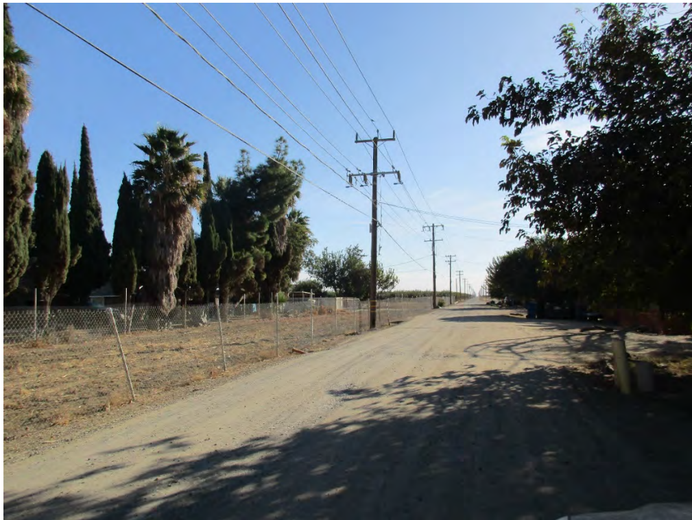
West Excelsior Avenue East of State Route 145
