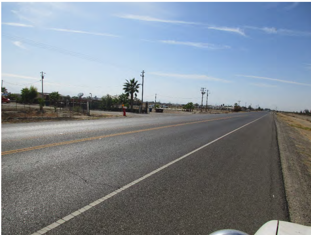
Looking Southwest Across State Route 180
