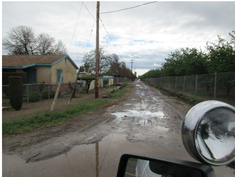
Southerly Dirt Road looking East – March 23, 2020
