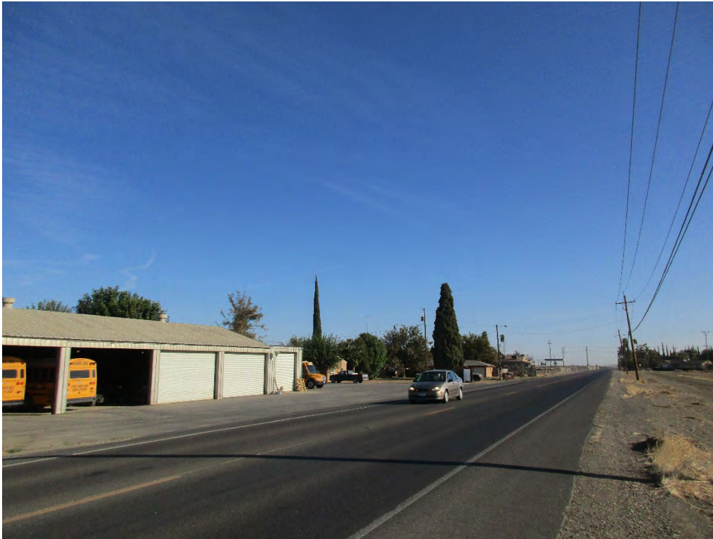
Northbound SR 145 – School Bus Facility to West
