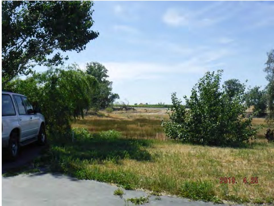
Private Ponding Basin looking West
