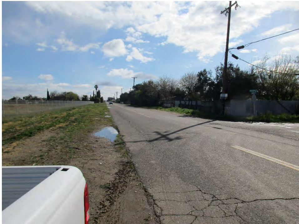
Church Avenue looking East – March 11, 2020
