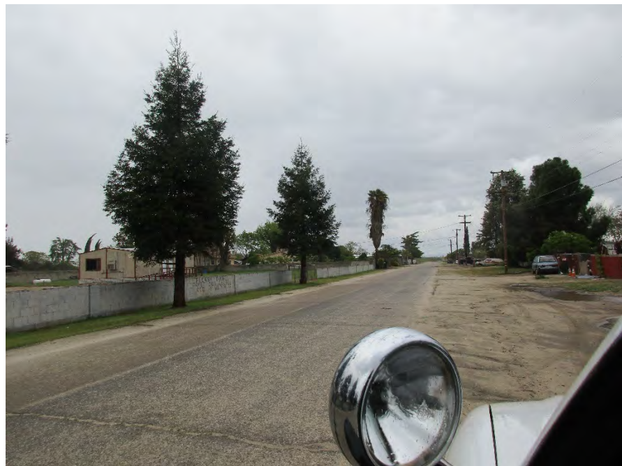
Fairbanks Avenue looking North from Central Avenue – April 6, 2020
