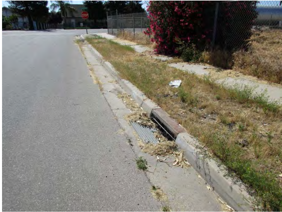
One of two Curb Inlets looking West
