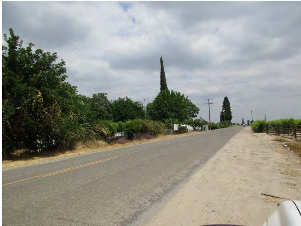
Church Avenue looking East
