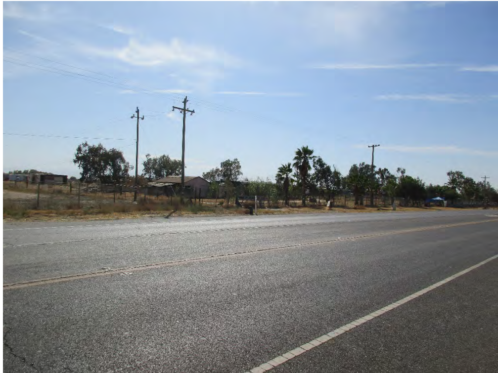
Looking Southwest Across State Route 180
