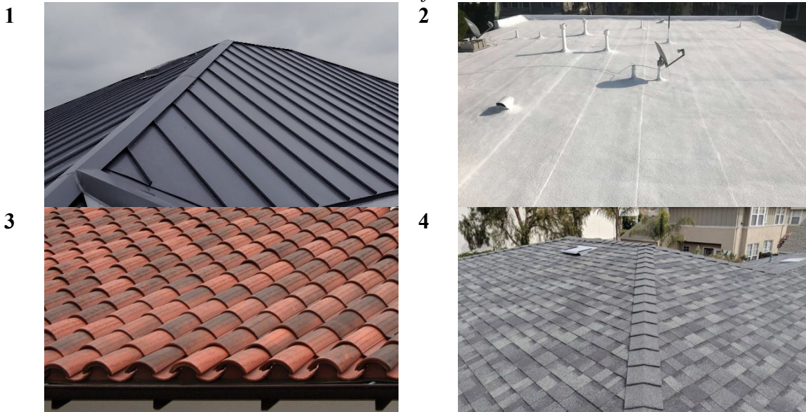
Figure 4-5 Allowable Roof Materials
