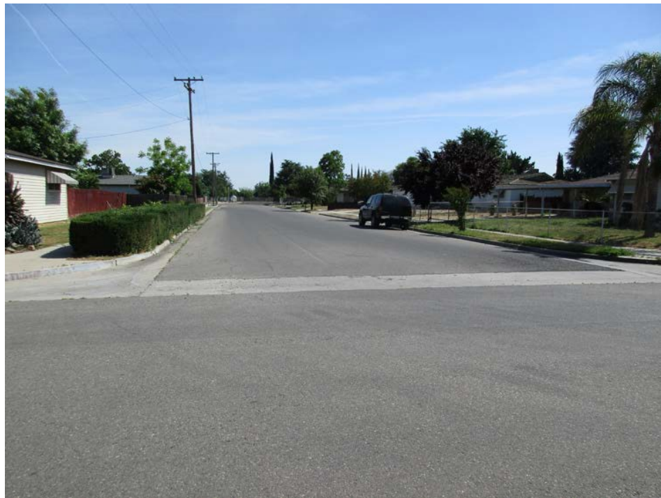
Typical Valley Gutter looking South
