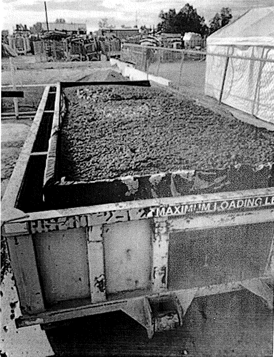
Photo 6 - Decanting Bin with Soil
