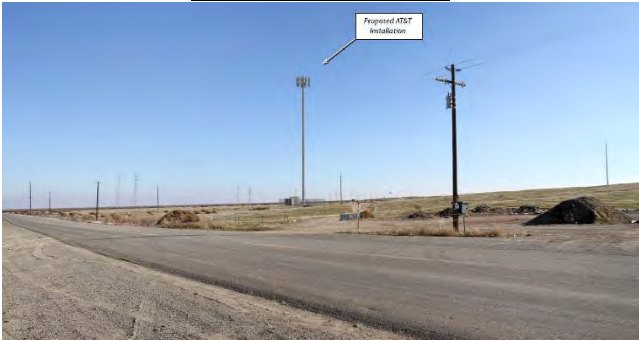
View from W Kamm Ave looking southeast
