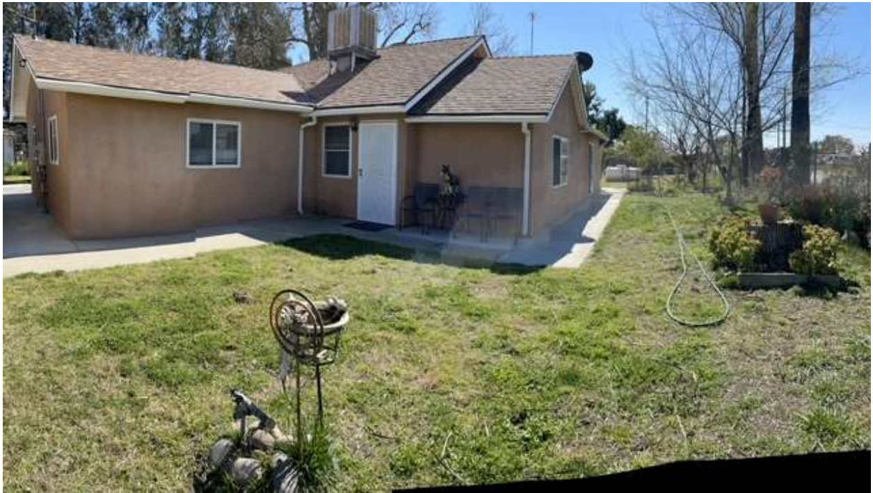
The House looking South
