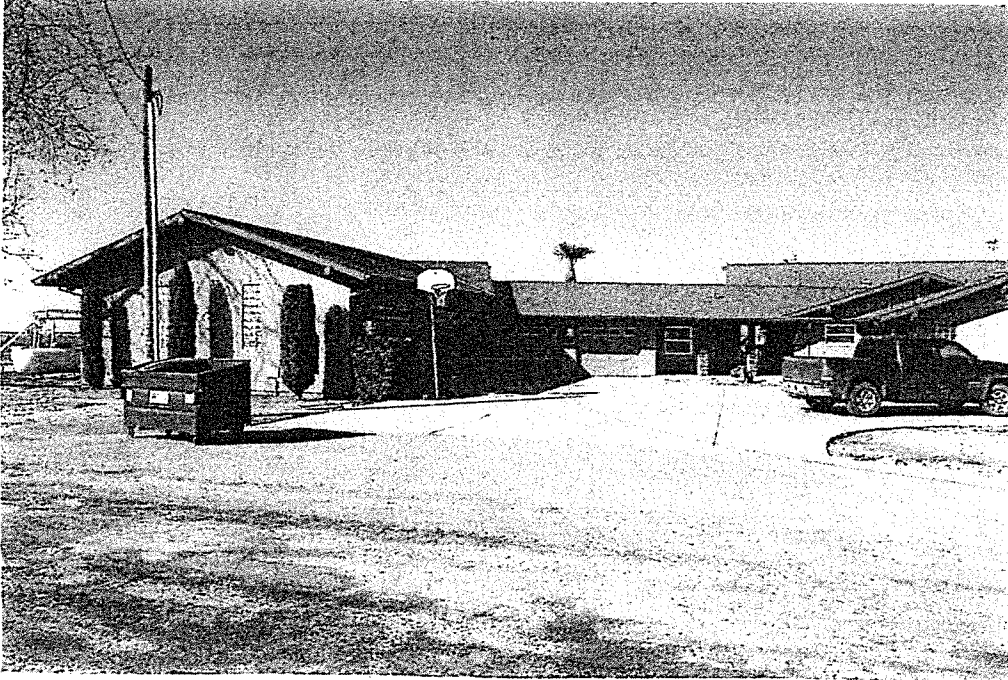
South View of Residence
