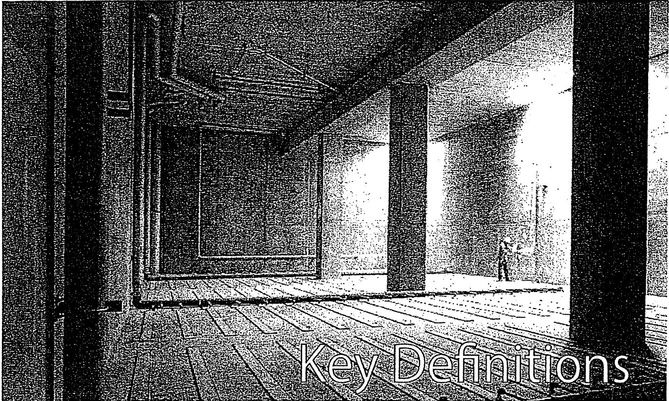
SPA III Water Recycling Facility 1.8 MGD Aeration Basin
