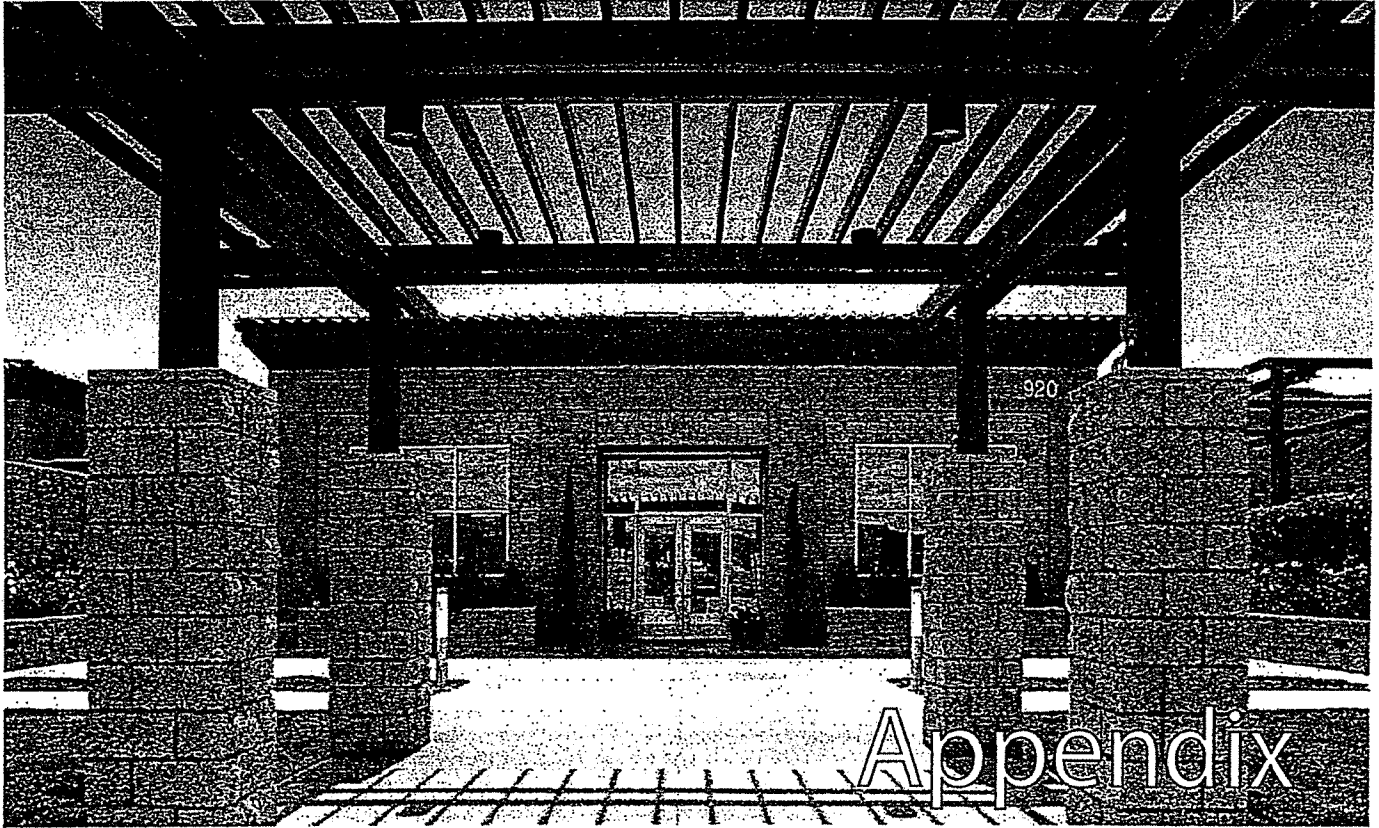
Santa Paula Water Recycling Facility 4.2 MGD Entrance
