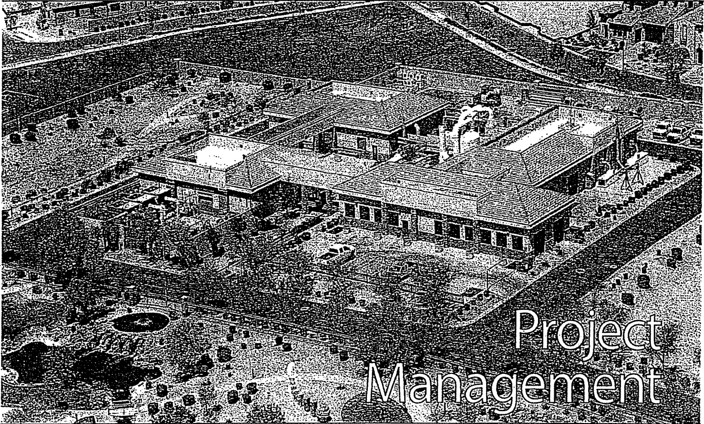
Palm Valley Water Recycling Facility 4.1 MGD Aerial View of SBR Facility
