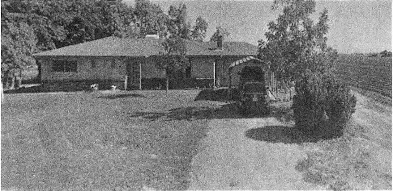
384 E Riverdale Ave APN 055-350-20S 1.57 AC Built 1977 2,280 FT from PIQ
