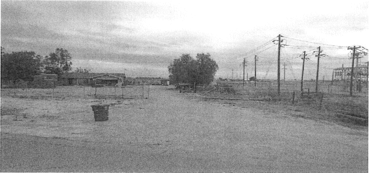
19890 S Elm Ave APN 055-220-42 1.23AC Built 1993
