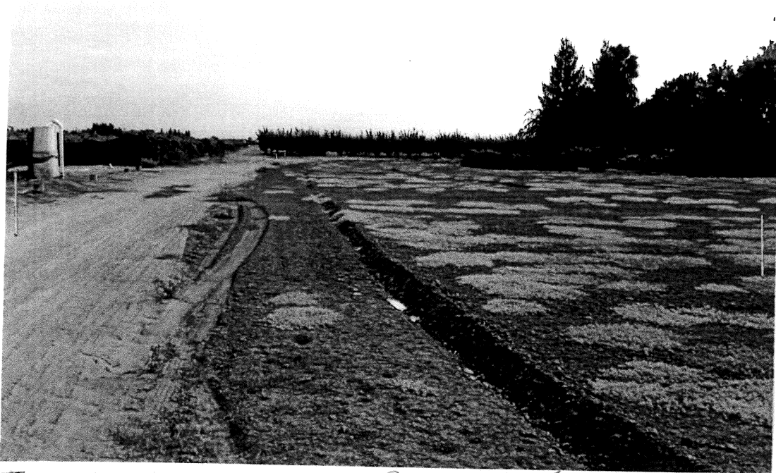
FROM: N/E CORNER OF PROPOSED 5 ACRE PARCEL LOOKING SOUTH TO END OF 20 ACRES.
