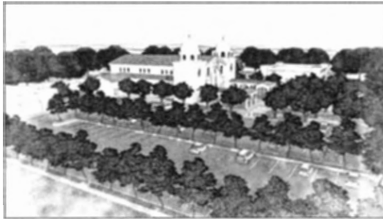
2 AERIAL VIEW LOOKING NORTHWEST
