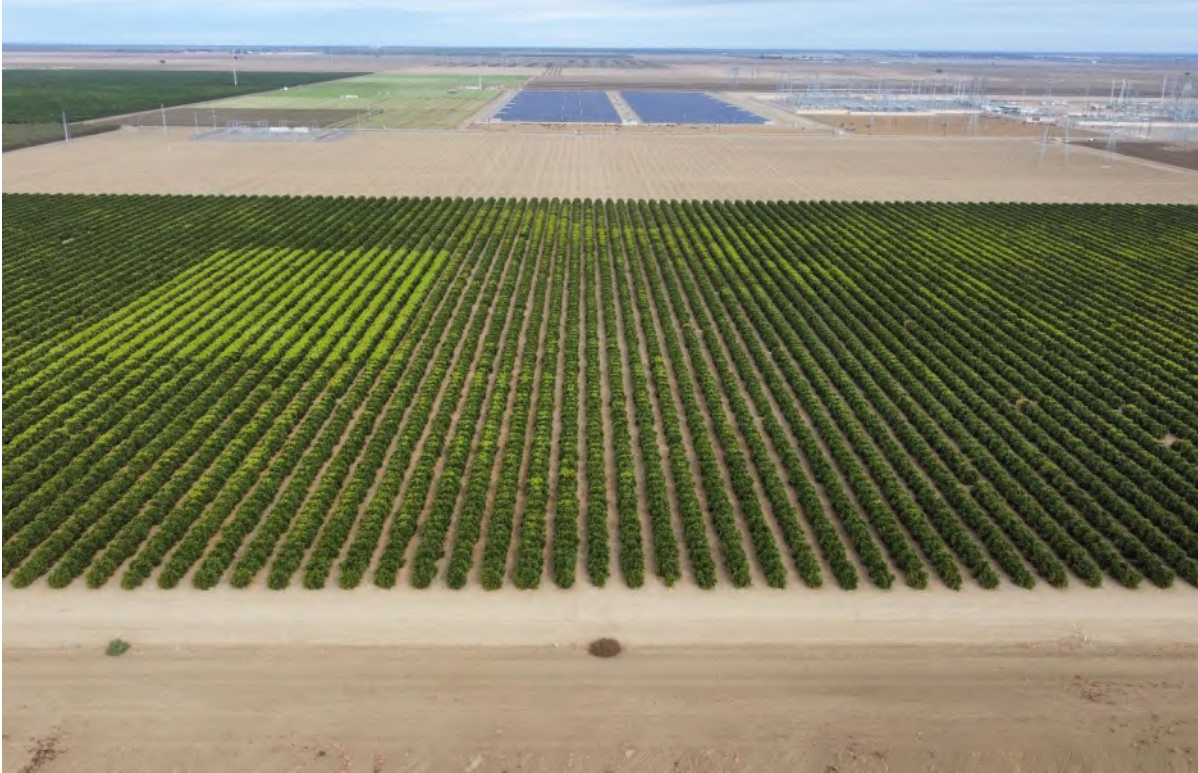
Photograph 1. Aerial view of Key 1 (APN 080-045-58S) looking north toward Gates Substation.
