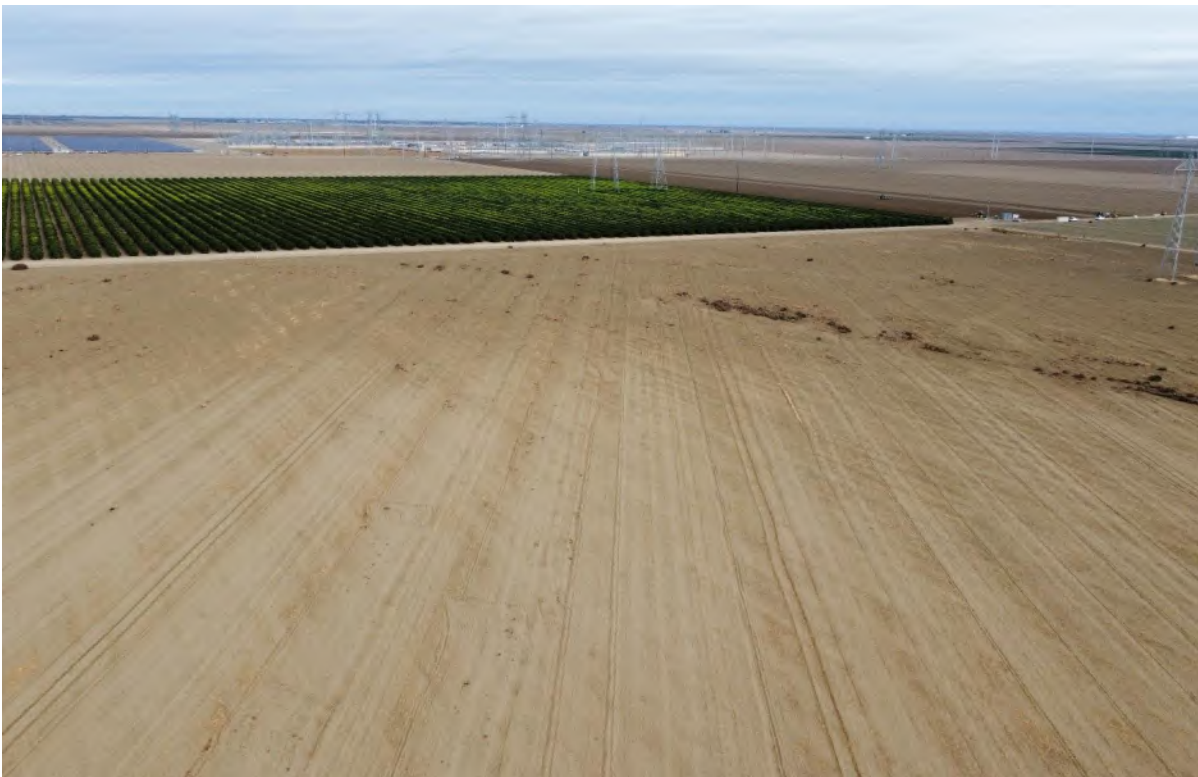
Photograph 2. Aerial view of Key 2 (APNs 080-045-36S and -37S) looking northeast toward Key 1 and Gates Substation.
