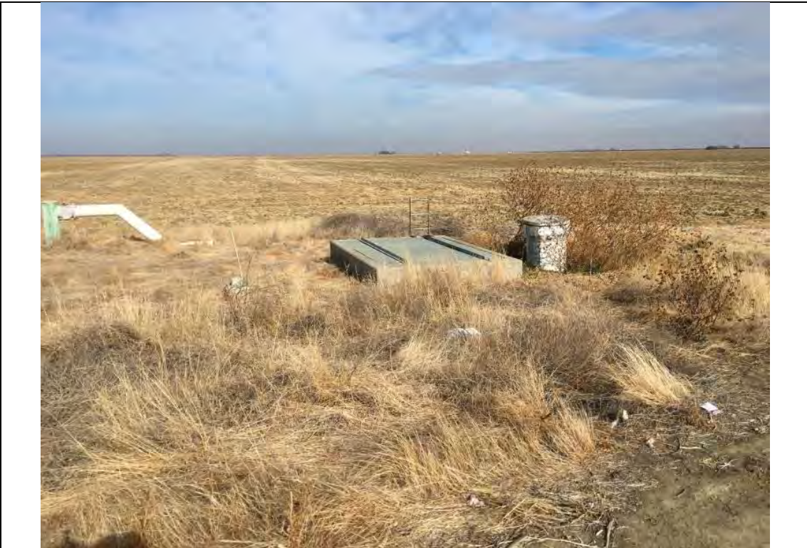
Photograph: 6 | View of underground water line access vault and irrigation piping.
