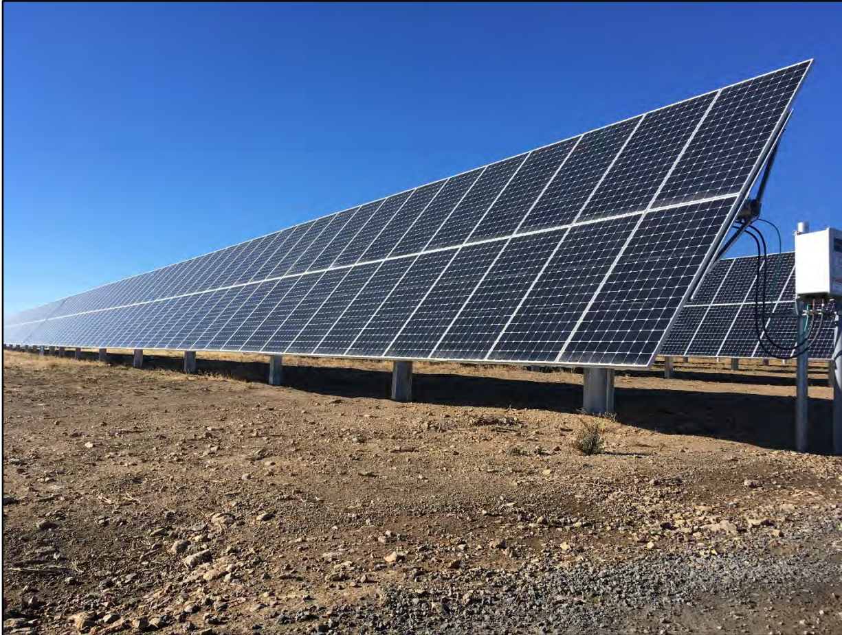
Figure 5. Typical Tracker Panel and Pier Design
