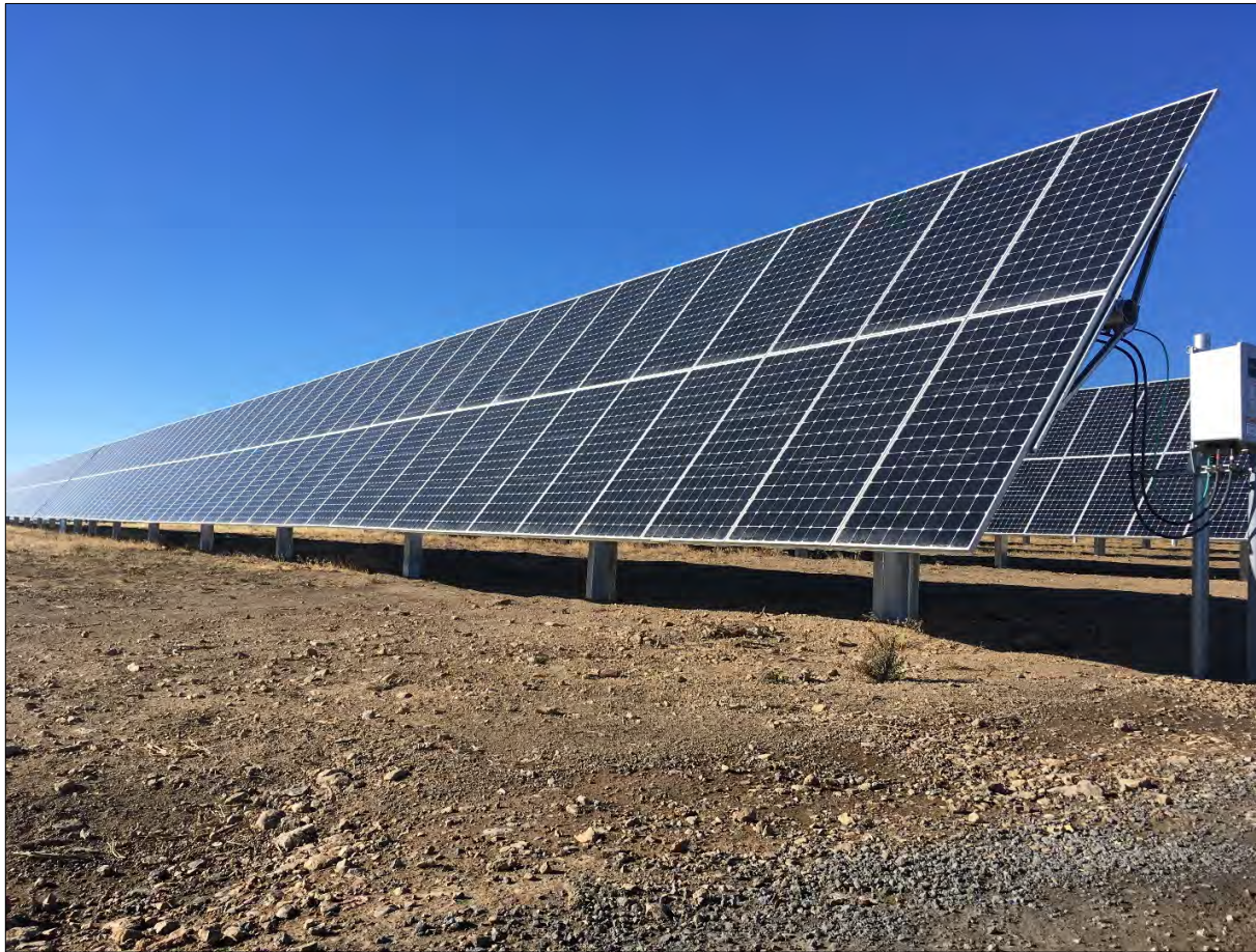
Figure 3. Typical Tracker Panel and Pier Design
