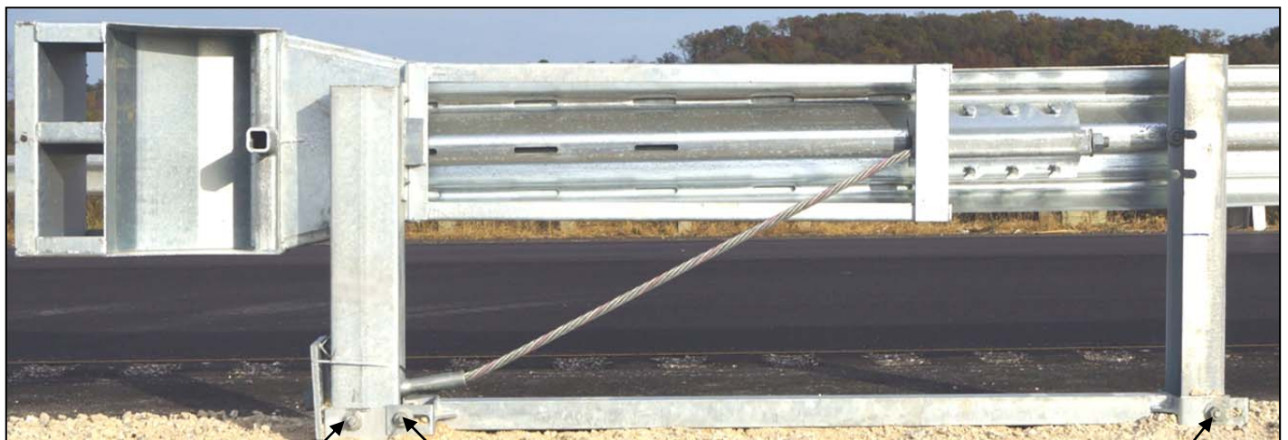
Post #1 Connection Detail
