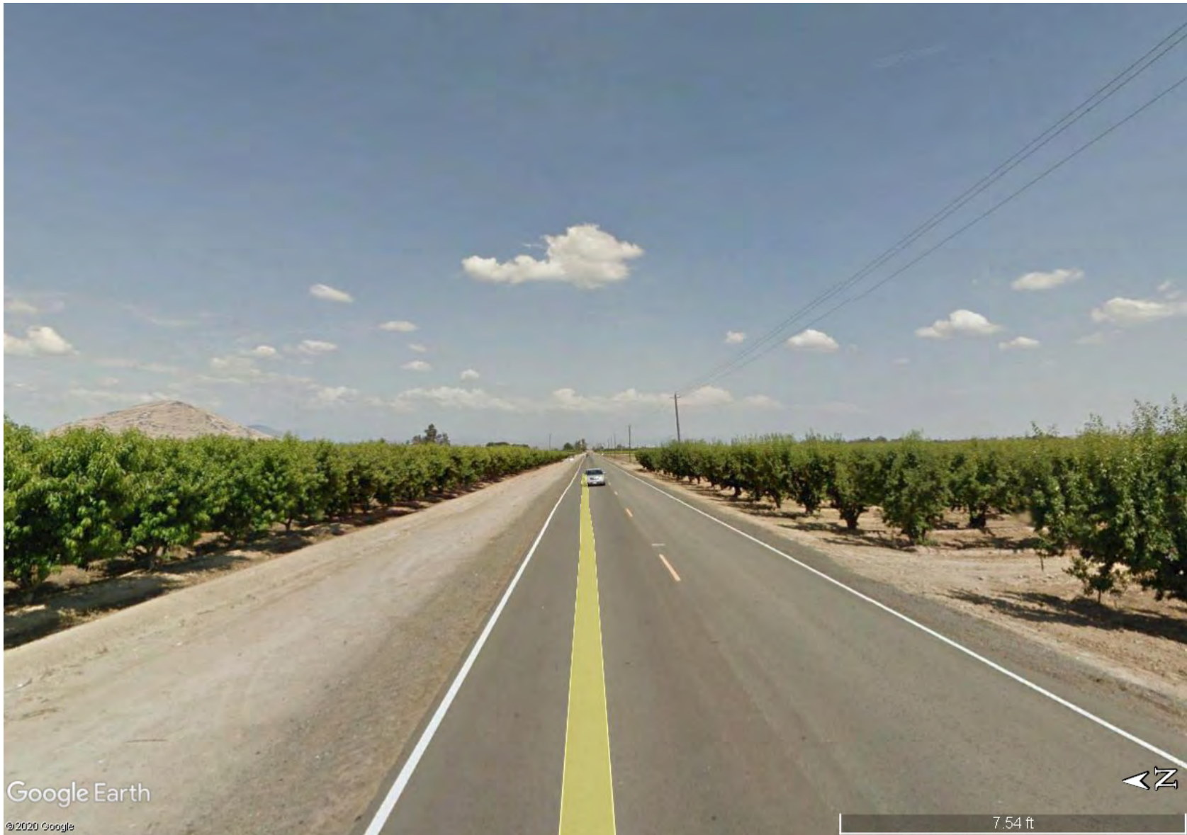
Figure 18 – E Goodfellow Avenue approximately 900 feet from the E Goodfellow Avenue and S Rio Vista Avenue intersection.
