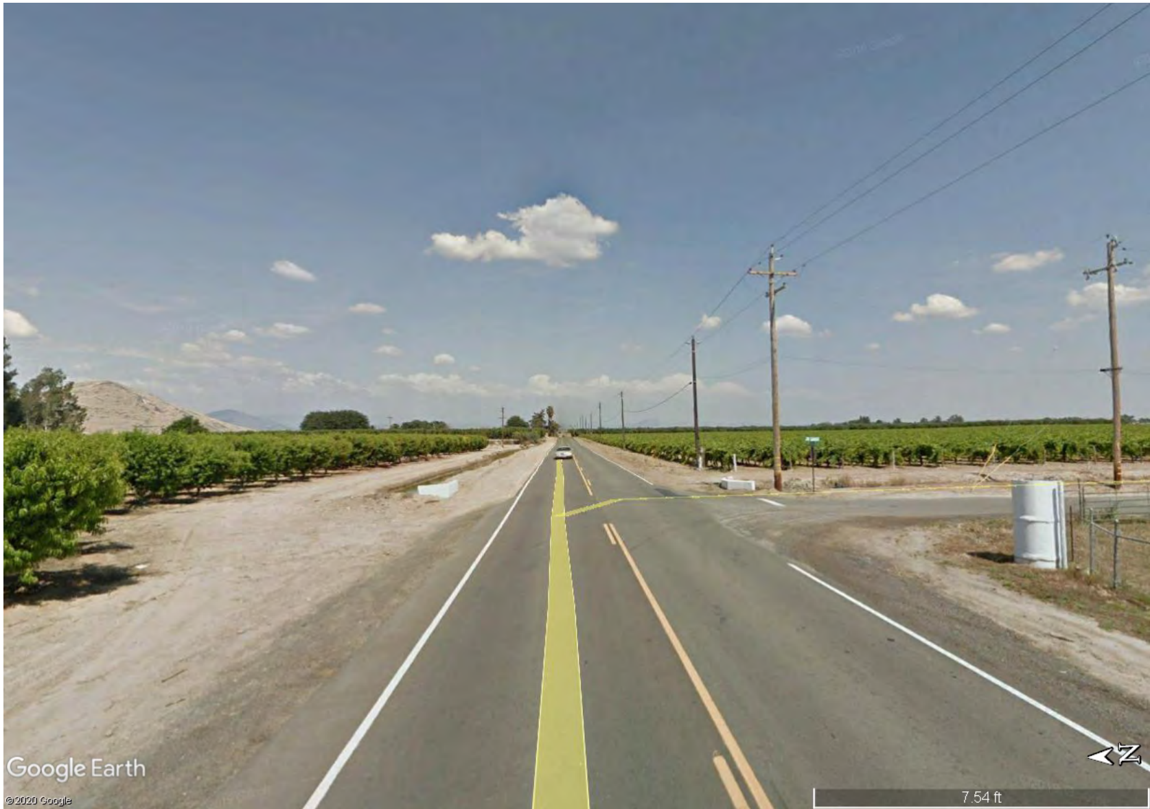
Figure 19 – E Goodfellow Avenue facing east towards ditch (left) and Jim Savage Road (right).
