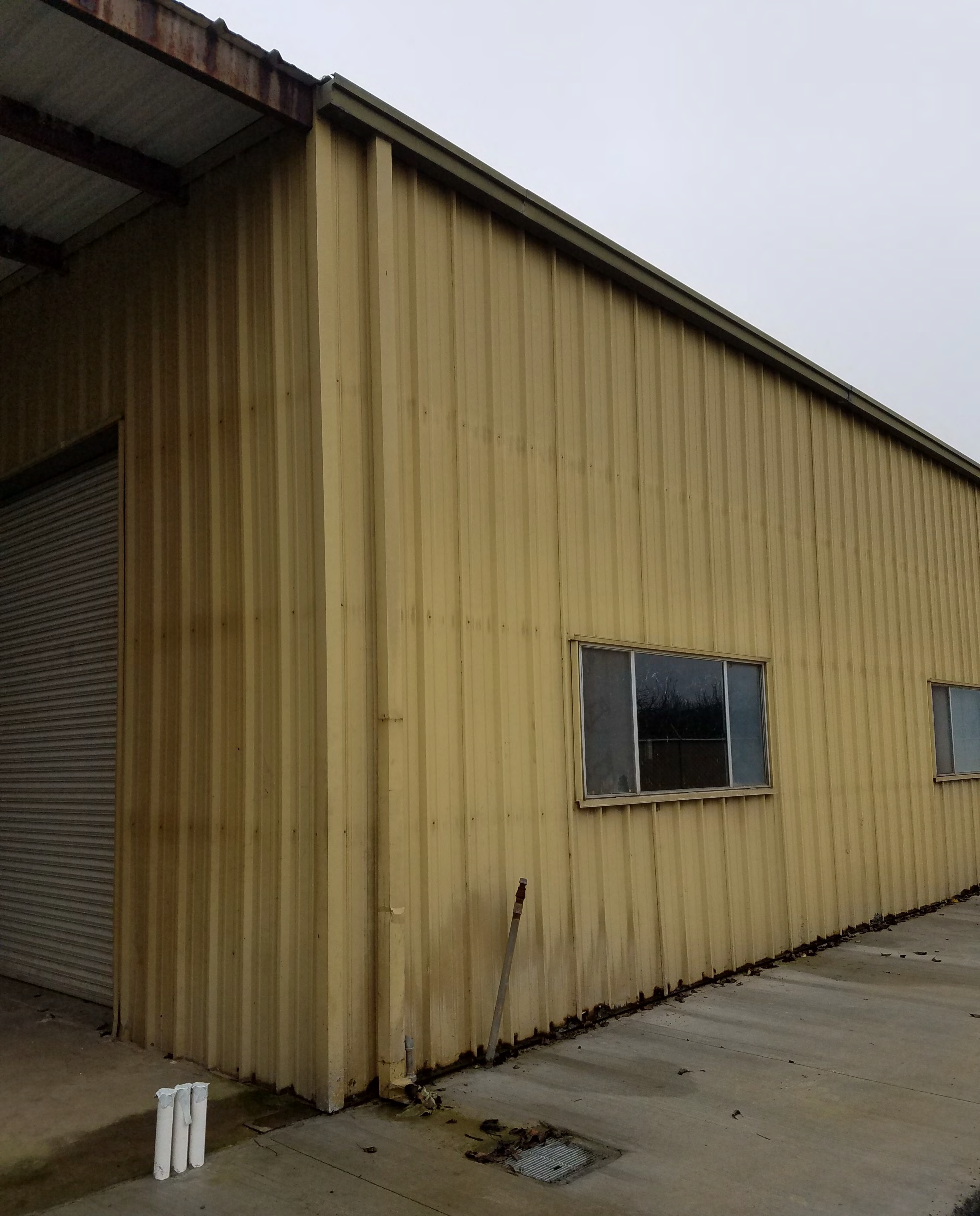
East & North side
