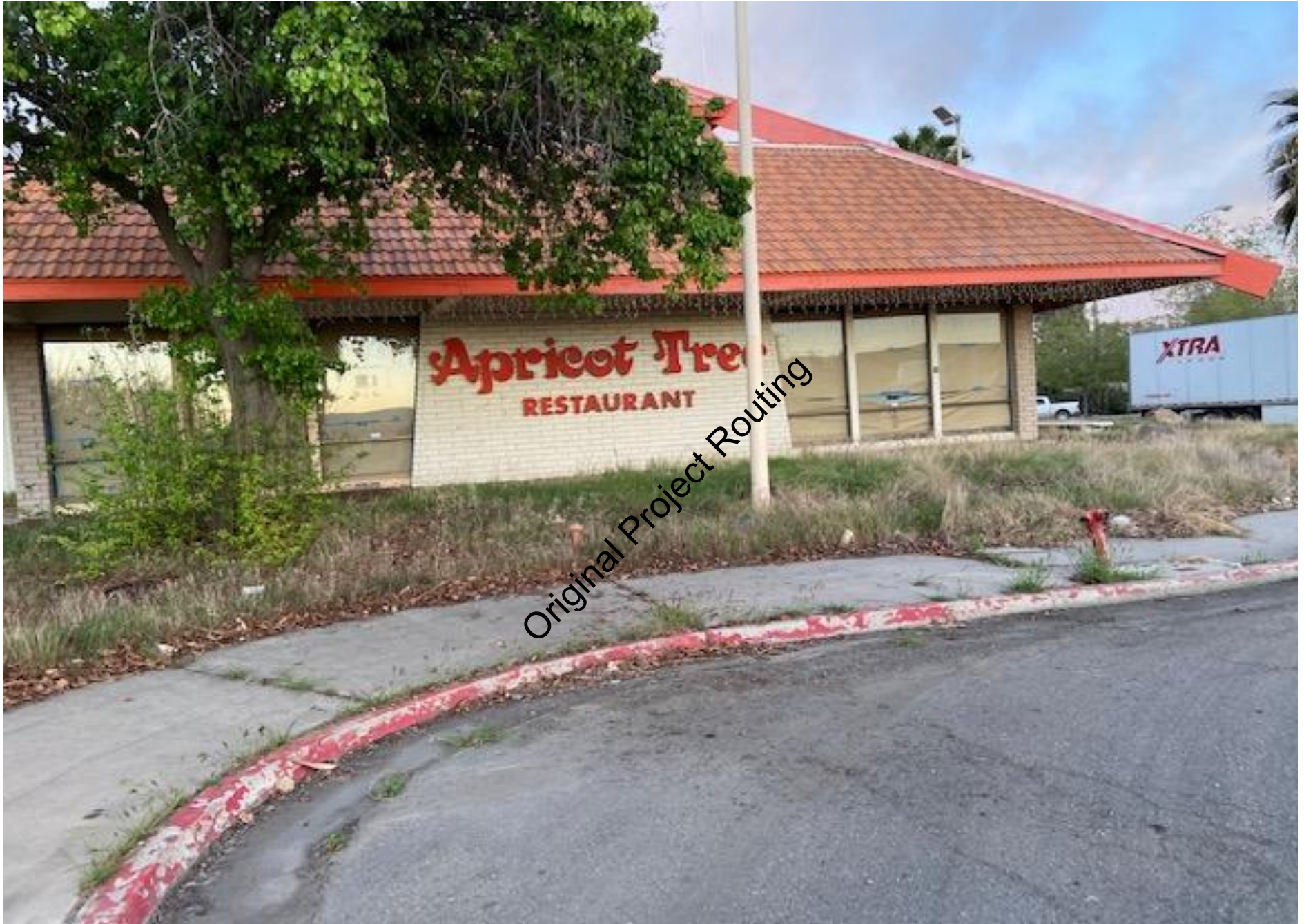
SIDE VIEW – WEST
