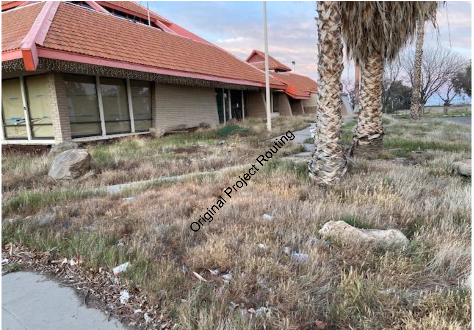
SIDE VIEW – WEST
