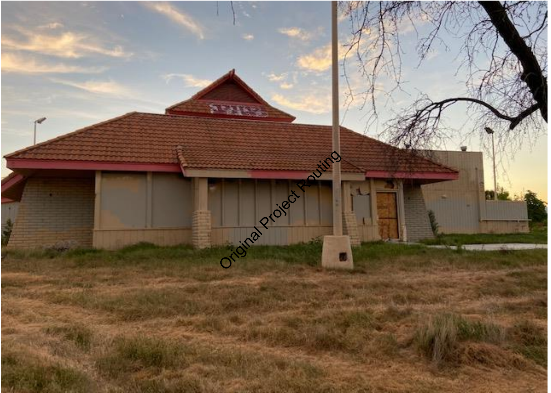
SIDE VIEW – EAST – FREEWAY SIDE
