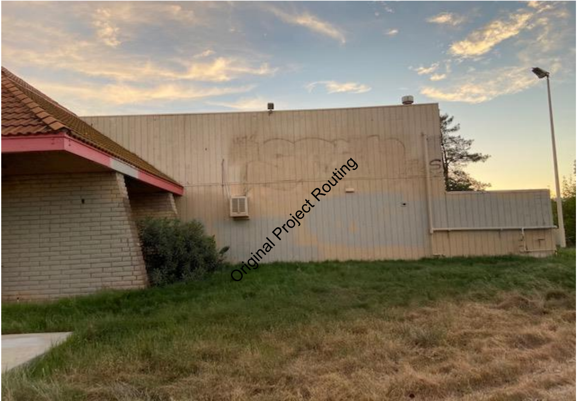
SIDE VIEW – EAST – FREEWAY SIDE
