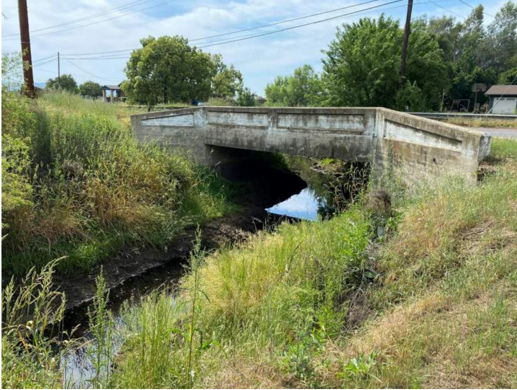
Figure 2 Photo taken on the northern side of the existing bridge.
