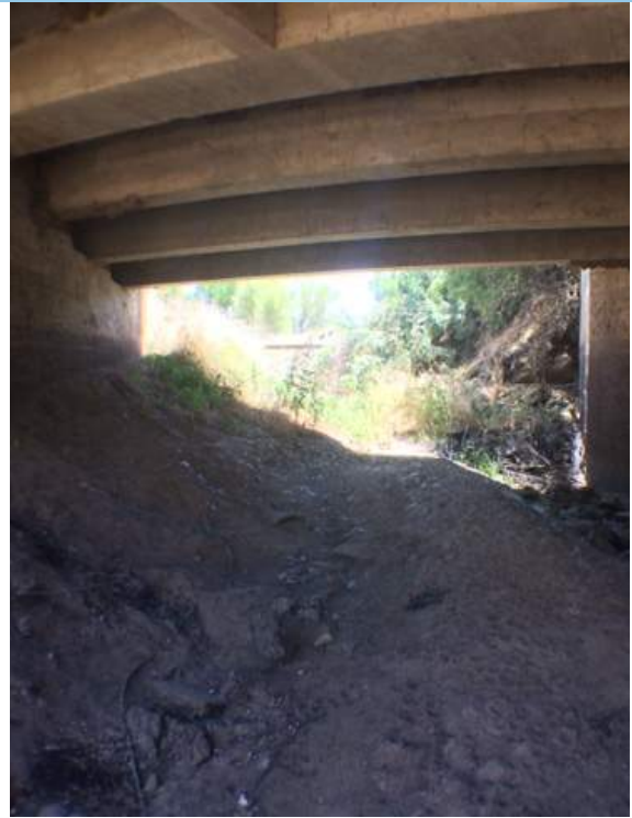
Photo #2. Travers Creek, underneath the bridge (facing south).
