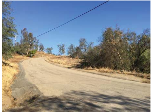
Photo #2 View of Ennis Road approaching Sand Creek Bridge, facing west.
