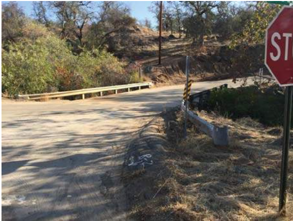
Photo #1 View of Sand Creek Bridge, facing north.
