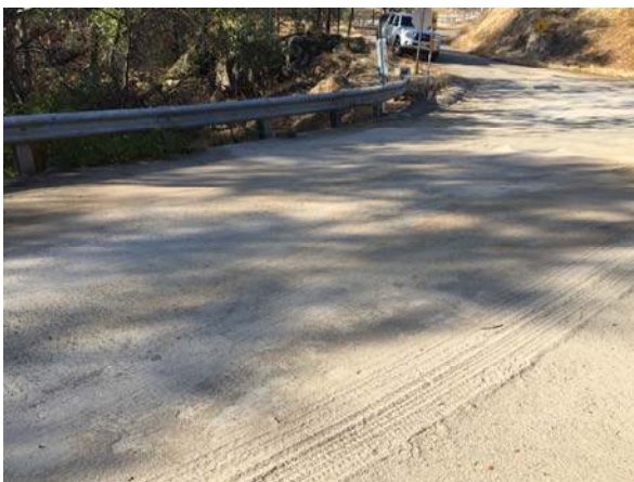
Photo #5 View of the south side of Sand Creek Bridge, facing south.
