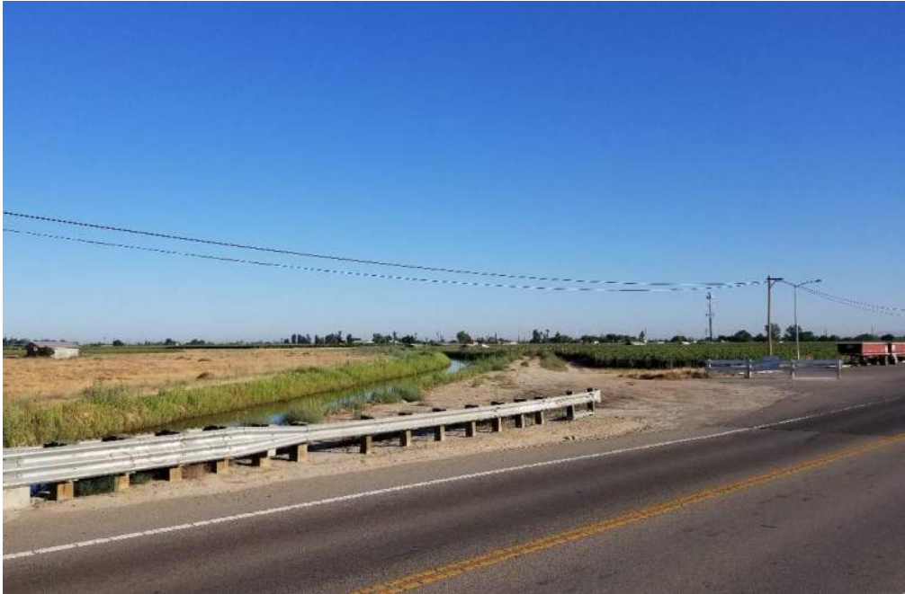
Figure 7 Additional example of a realigned access road with a paved driveway.
