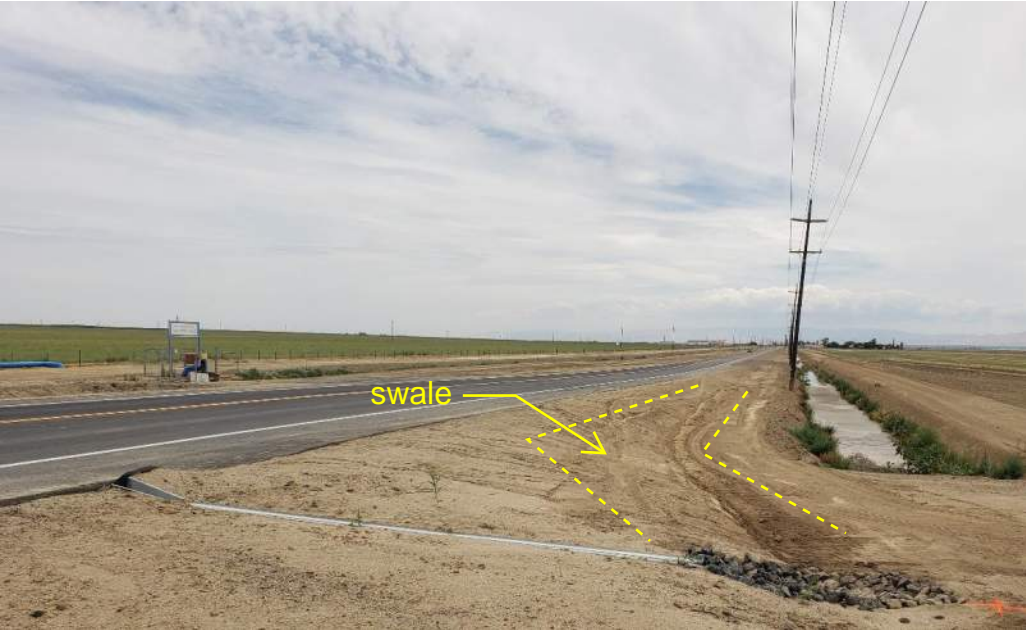
Figure 10 Additional drainage swale with a shallow depression located near a small drainage canal. Outside Canal Bridge Replacement Project on Russell Avenue.
