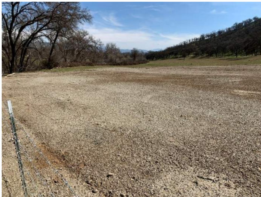
Figure 3 Temporary construction yard after construction. Watts Creek Bridge Replacement Project.
