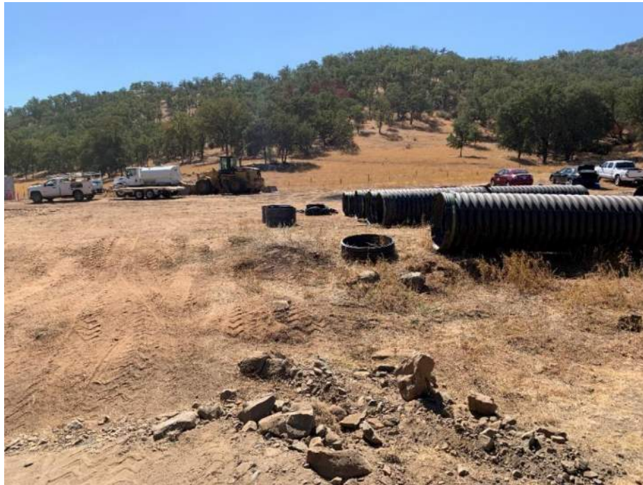
Figure 2 Temporary construction yard during construction. Watts Creek Bridge Replacement Project.
