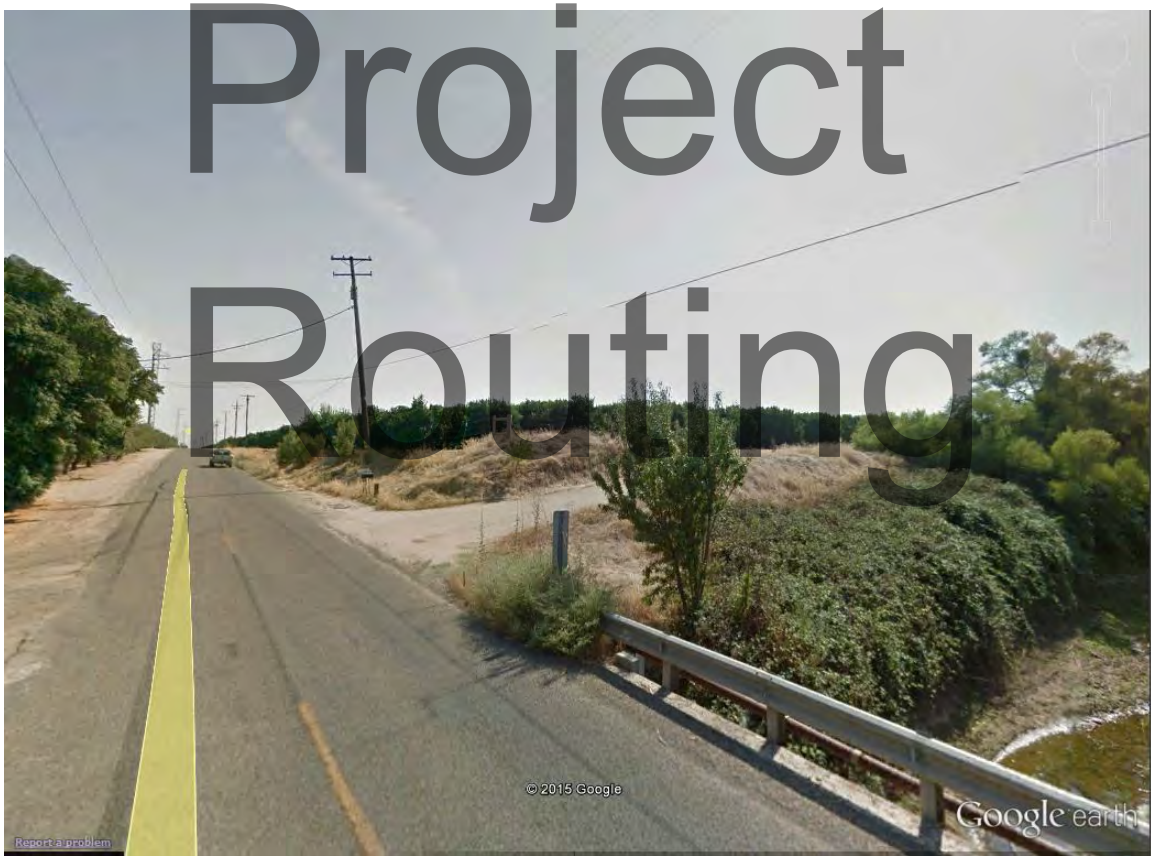
Access road on southwest corner of Fresno Canal
