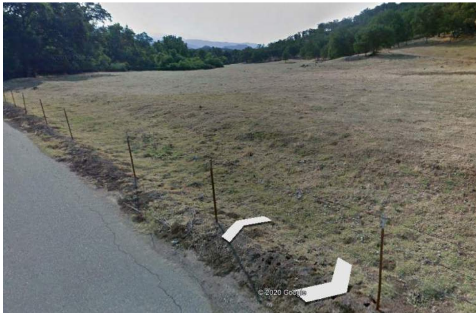
Figure 1 Temporary construction yard prior to the start of construction. Watts Creek Bridge Replacement Project.
