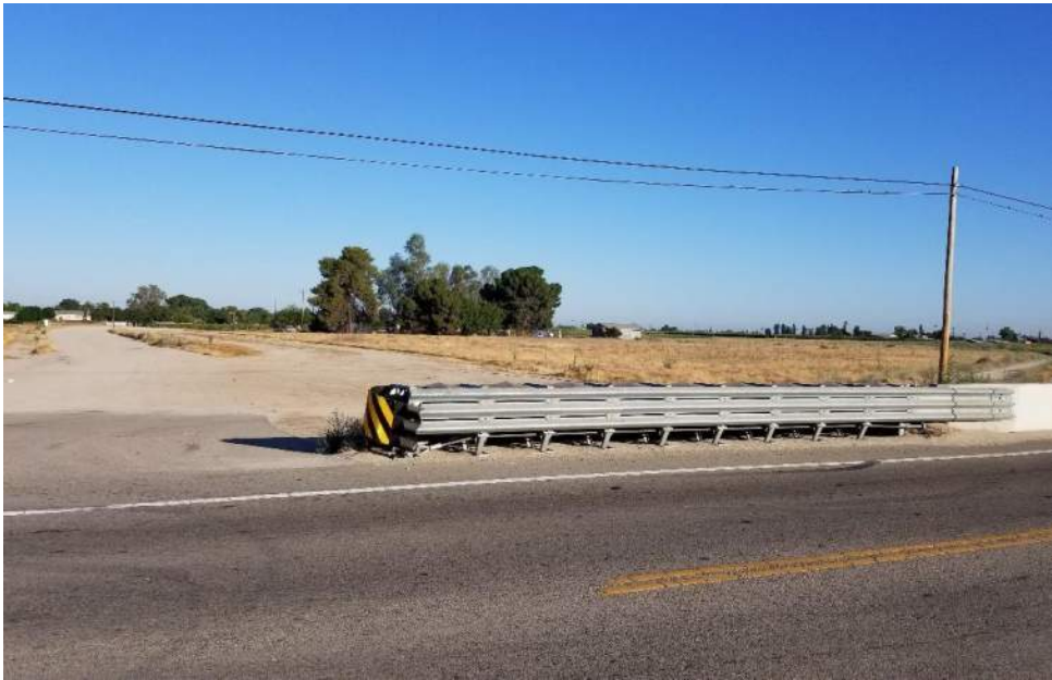
Figure 8 Additional example of a realigned access road with a paved driveway.
