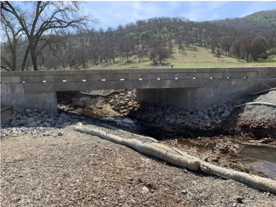
Figure 15 Side view of the completed bridge and project site at Watts Creek on Watts Valley Road.
