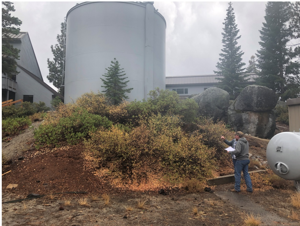
Proposed location of generator on the property
