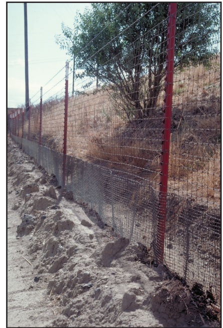
Figure 3. Small mesh wire fence.
