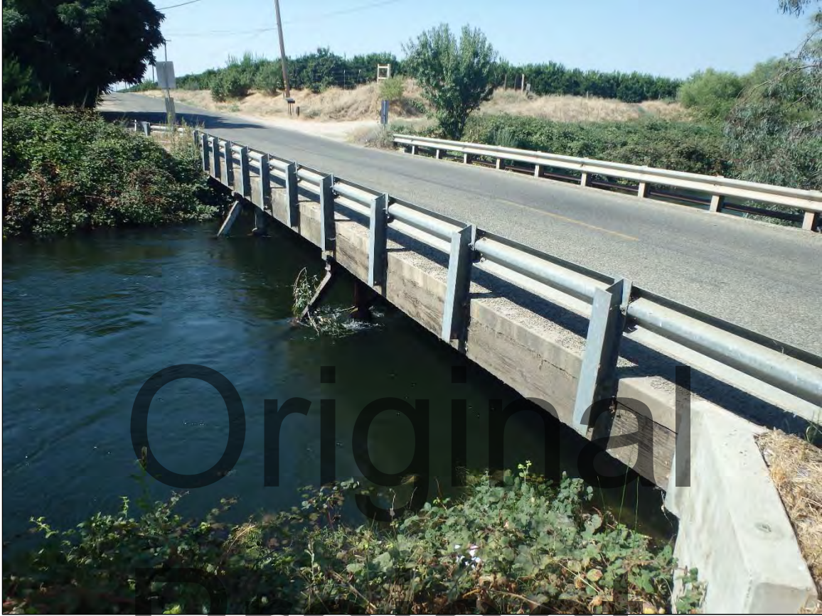
Figure 5 Overview of Bridge 42C0496 from northeast corner, facing southwest.
