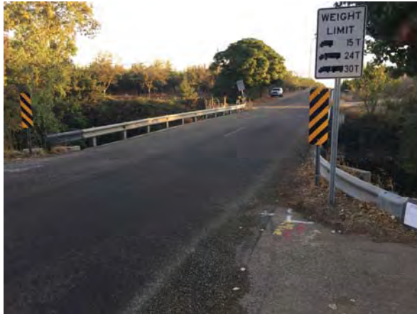
Photo #1 View of the Fresno Canal Bridge, facing south.
