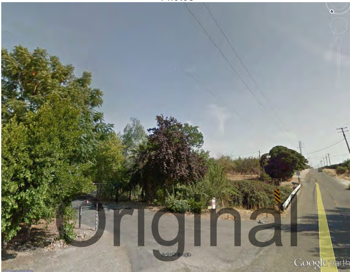
Driveway on northeast corner of Fresno Canal
