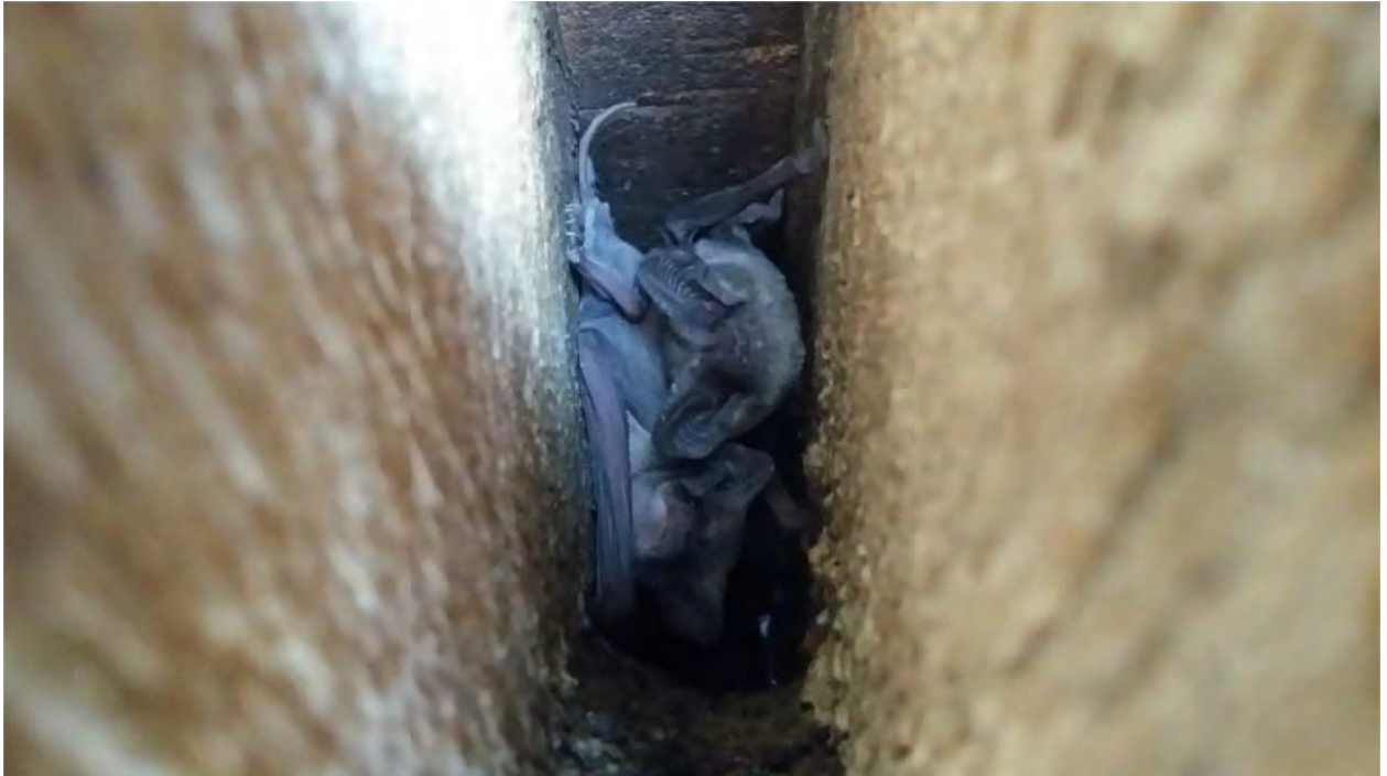
Photo 7: Mexican free-tailed bats under existing bridge. Free tail clearly visible.
