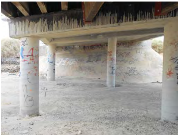
Photo #5 View below Jacalitos Creek Bridge, facing east.
