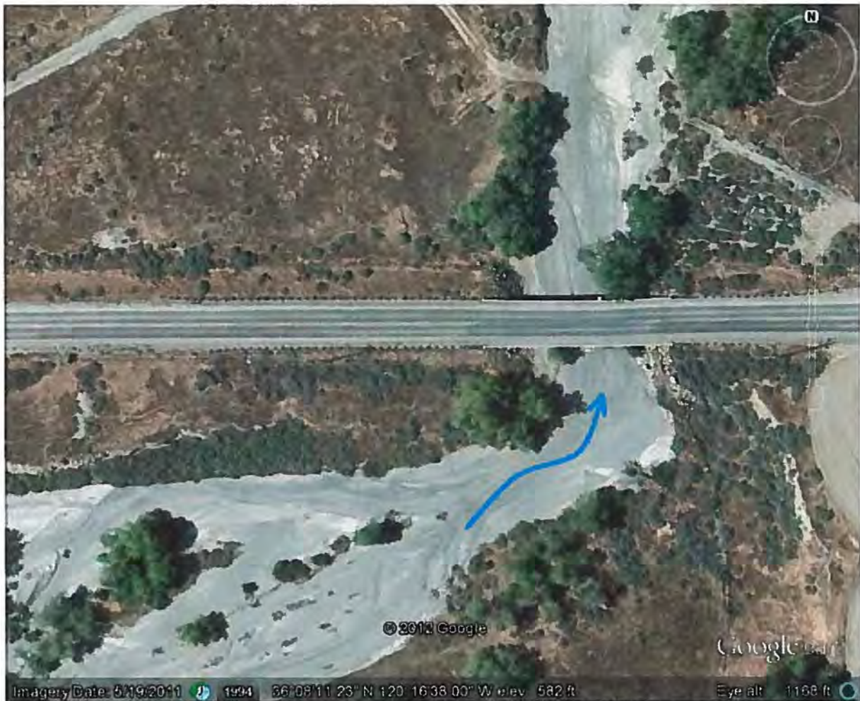
Figure 1: Aerial View of existing Jacalitos Creek Bridge, Br. No. 42 0072.
