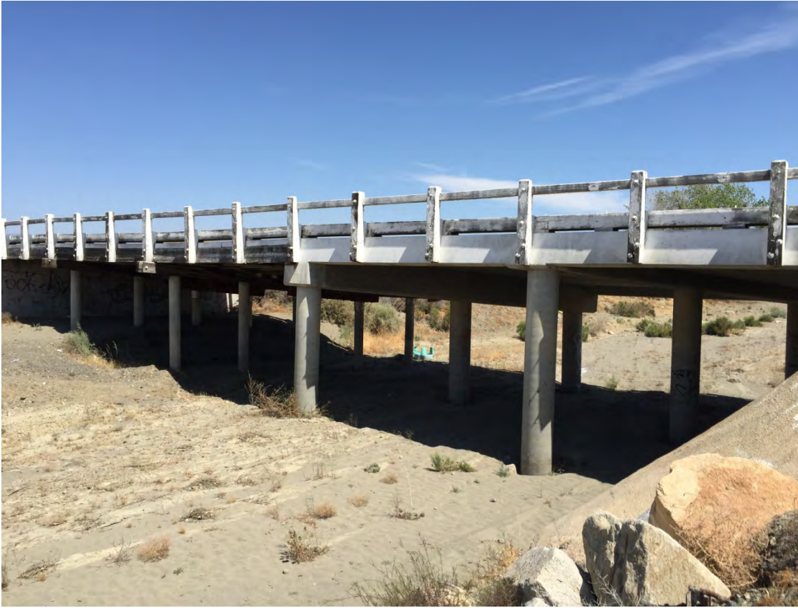
Photo 1. Existing Jacalitos Creek Bridge
