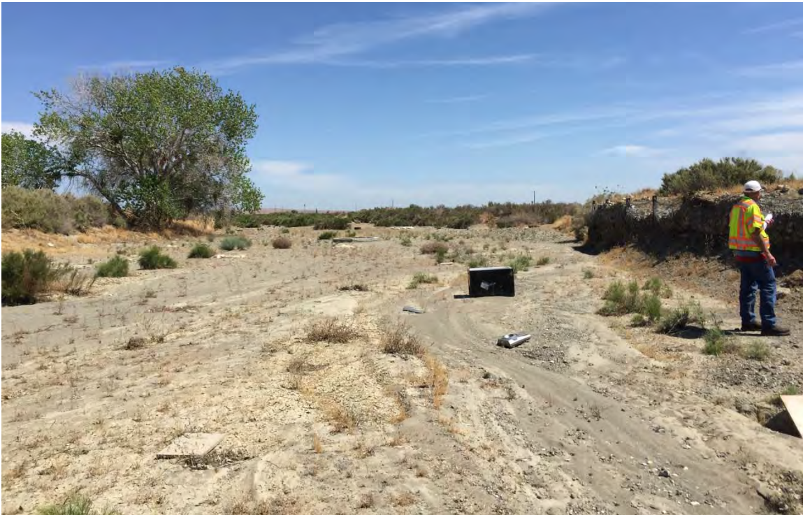
Photo 3. Jacalitos Creek Channel (Downstream of W Lost Hills Road)
