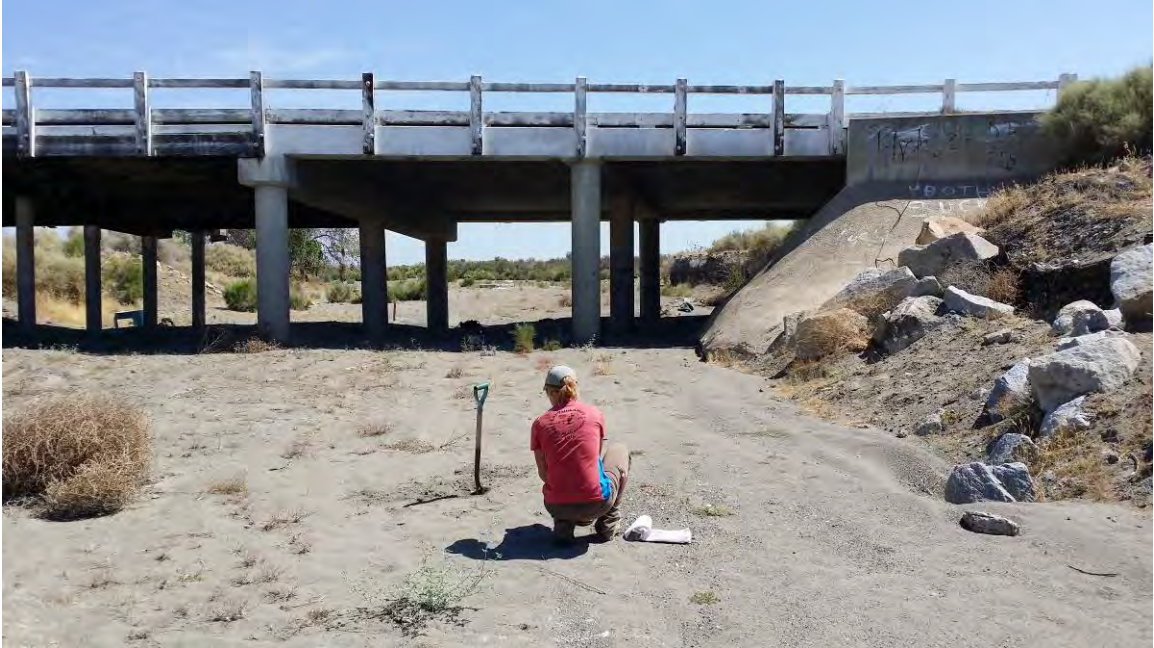
Photo 1. Sample Point 1 within OHW of Jacalitos Creek channel.
