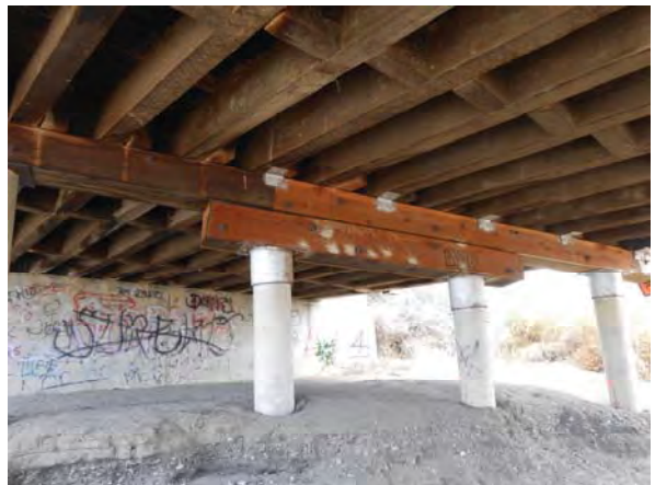
Photo #6 View of the bottom of Jacalitos Creek Bridge, facing northwest.
