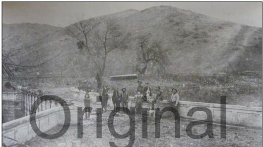
**Image 1.** New AID Main Canal headgate and bridge on North Frankwood Avenue, as constructed in 1914, camera facing southwest. <sup>17</sup>
