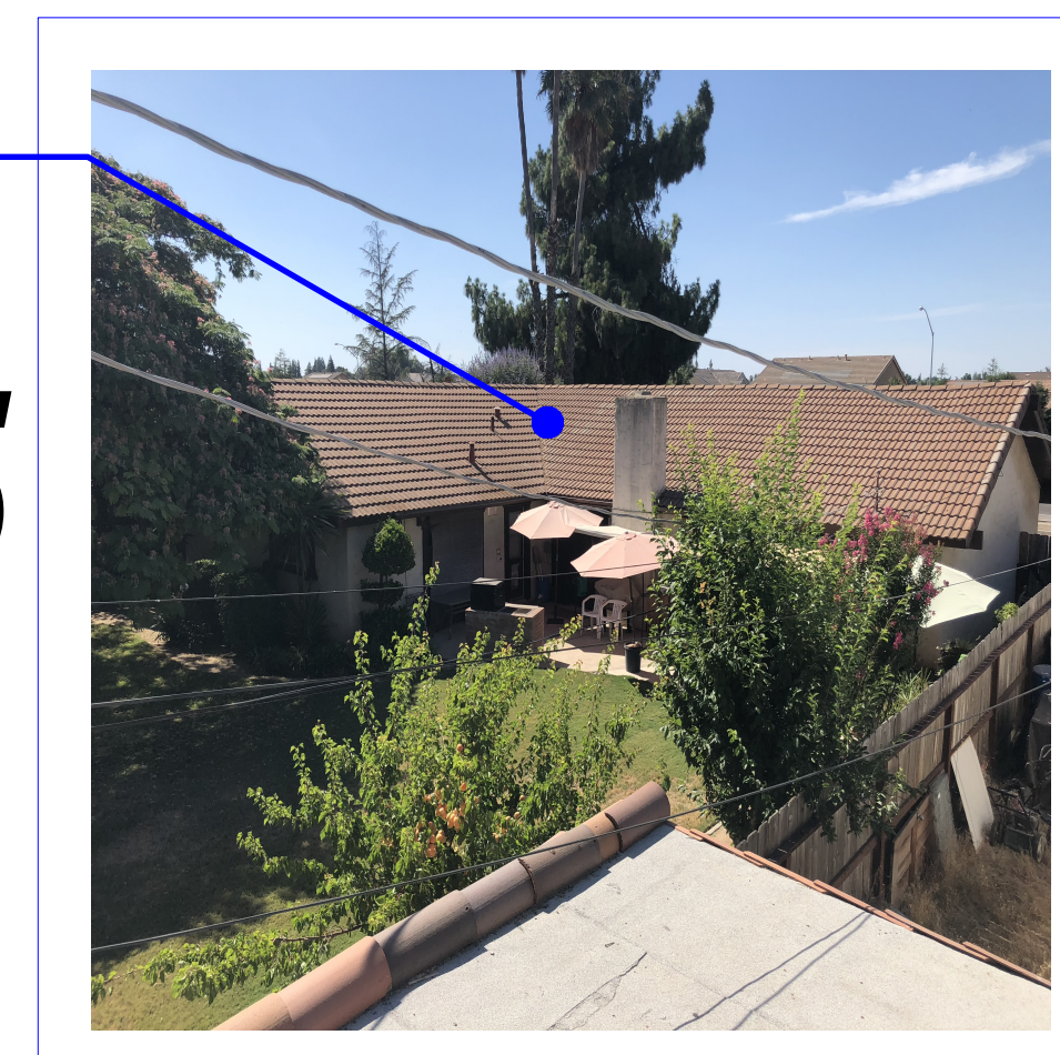
VIEW FROM ROOF OF ACCESSORY TOWARD NORTHWEST : house and landscape of neighbor rear yard
