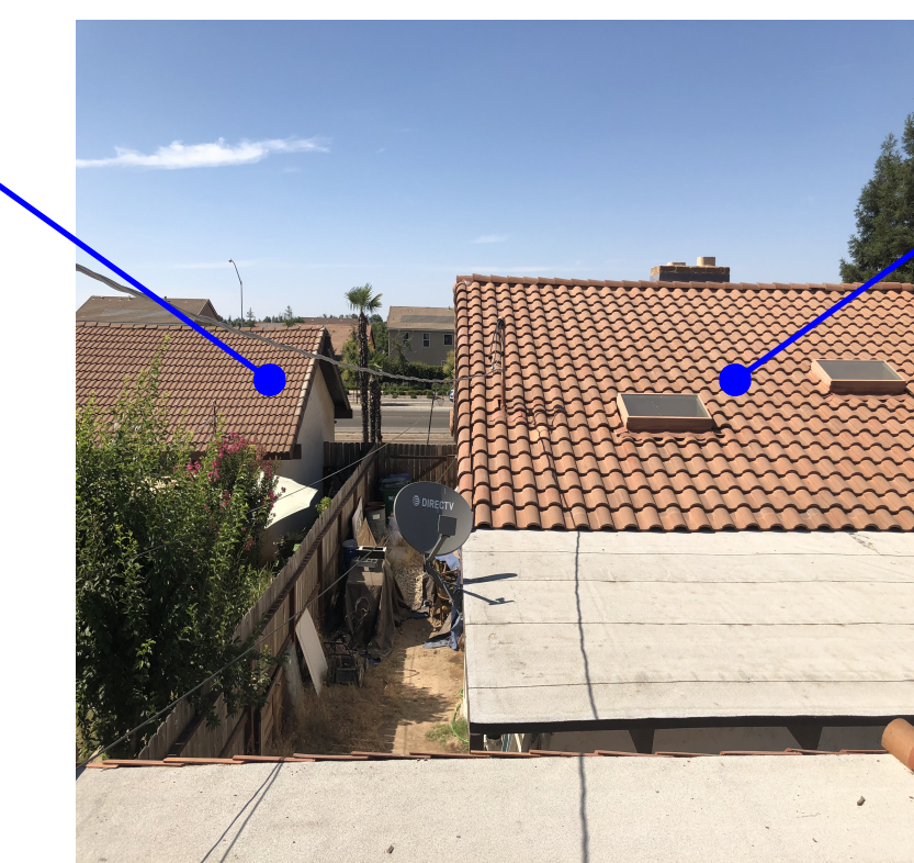
VIEW FROM ROOF OF ACCESSORY TOWARD NORTH applicant and adjacent roofs
