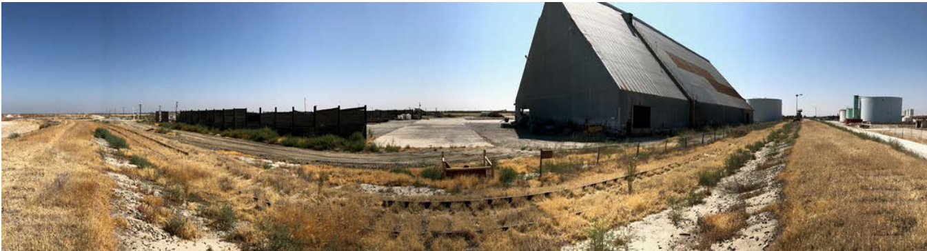
From East Site Boundary Looking East
