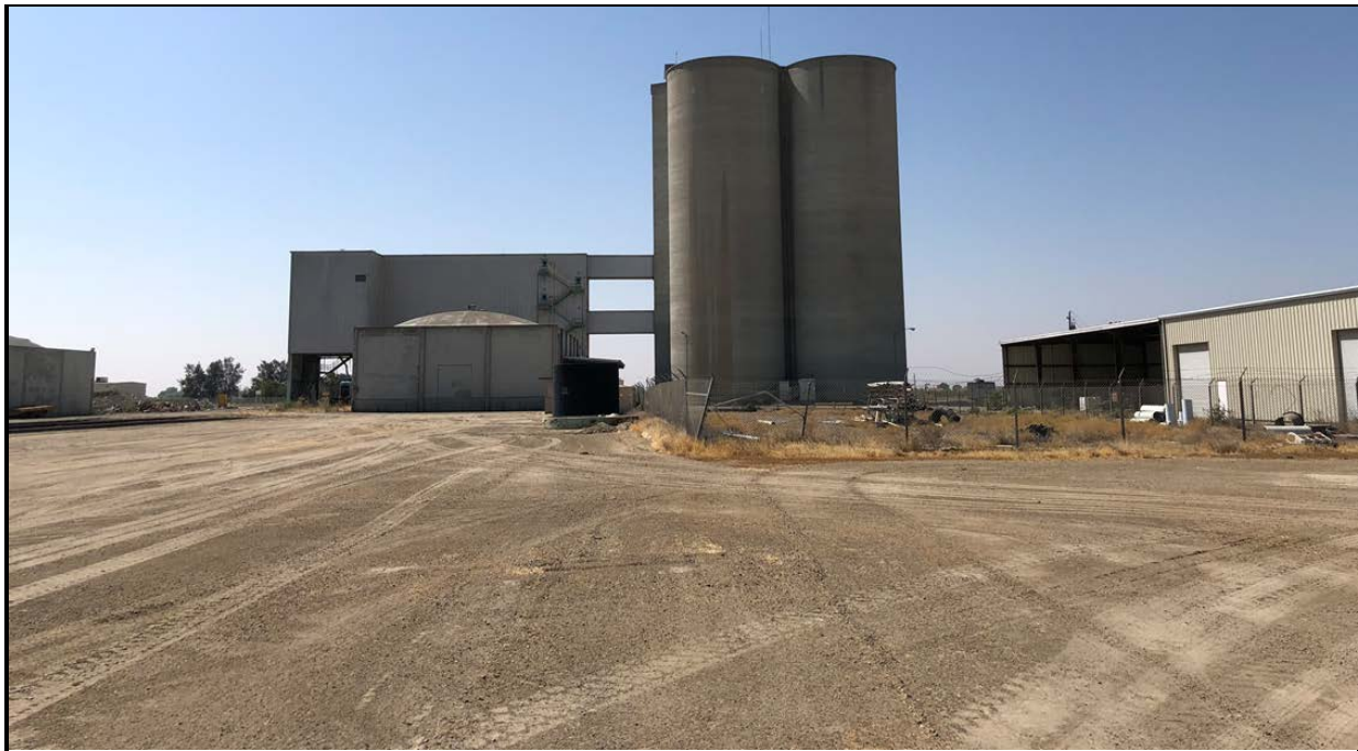
Figure 3-4. View of Storage Pile Area Looking South at Storage Silos
