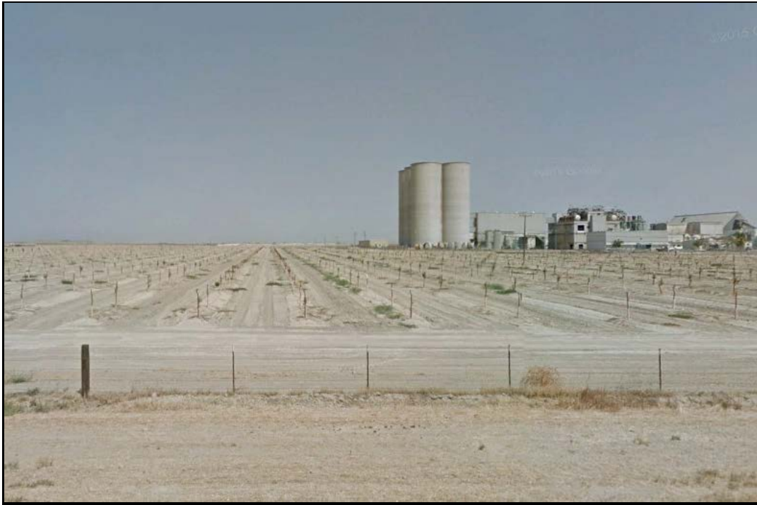
Figure 3-3. View of Existing Site from SR 180 / W. Whitesbridge Avenue
