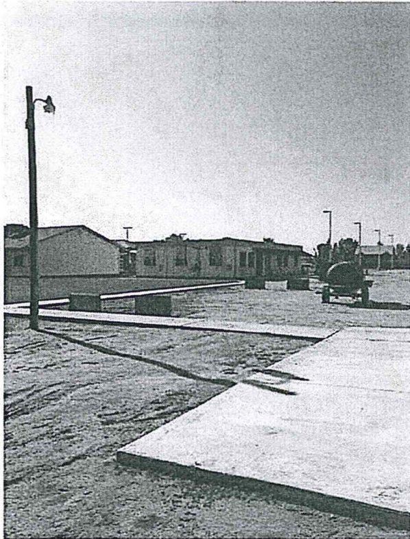
VIEW LOOKING SOUTH-WEST FROM EXISTING STORAGE BUILDING TOWARDS EXISTING OFFICES TO BE REMOVED
