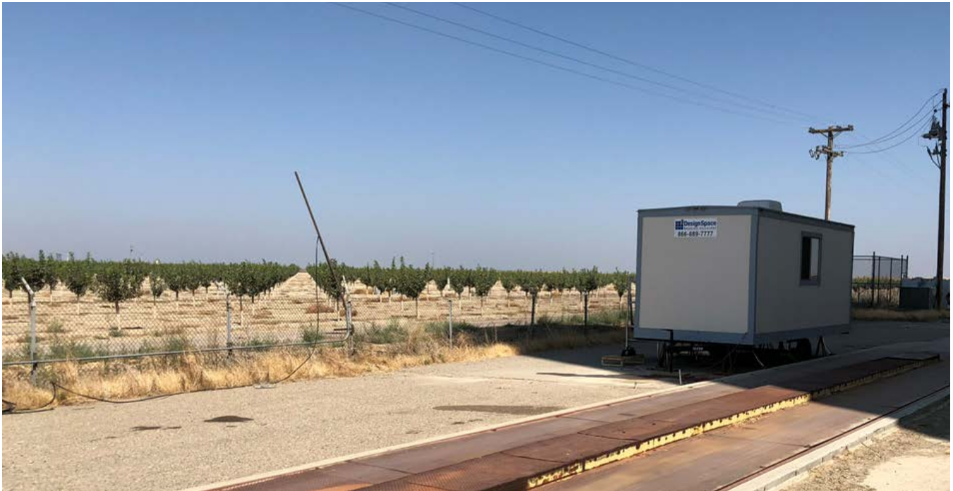
Figure 3-6. View of Existing Trailer for Office/Scale House
