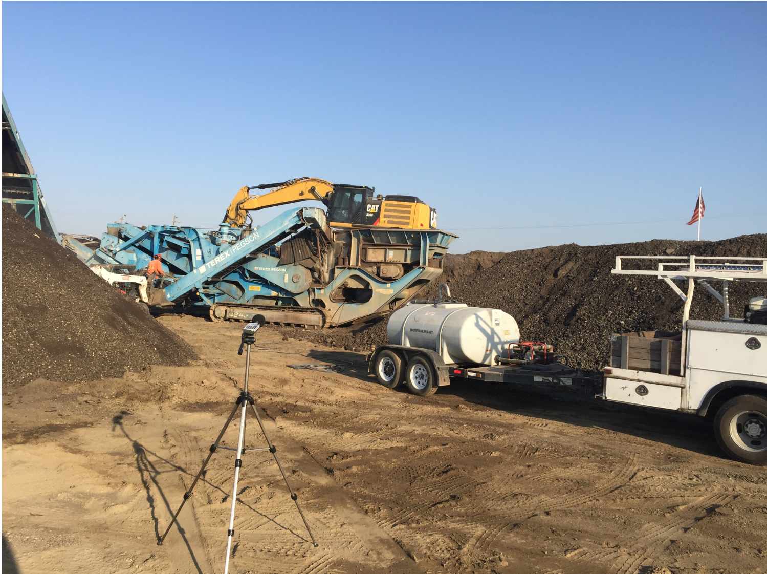
FIGURE 3: REFERENCE NOISE MEASUREMENTS, NOVEMBER 1, 2017
