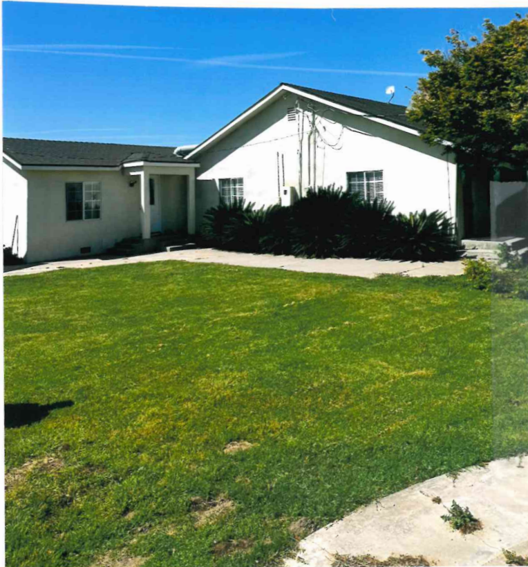
NORTH SIDE OF HOME
