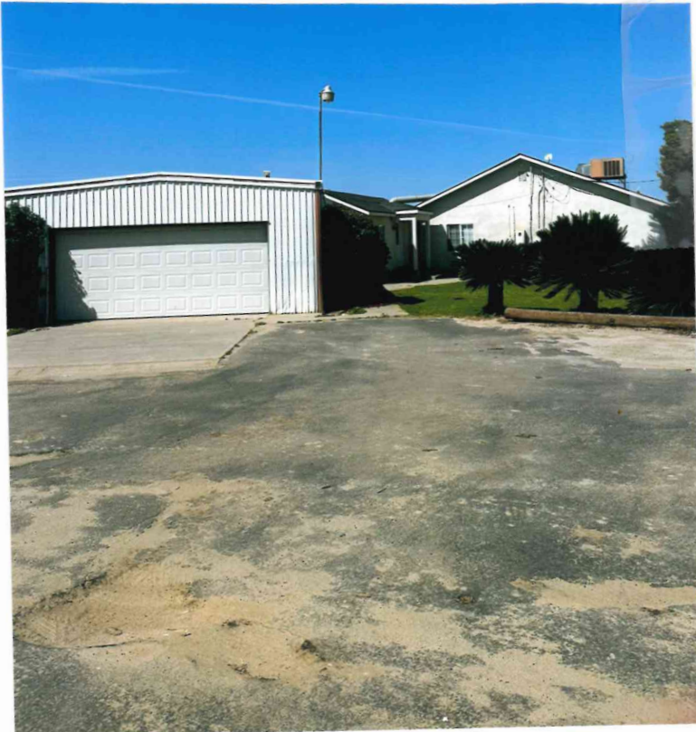
FACING EXISTING HOME - NORTH EAST
