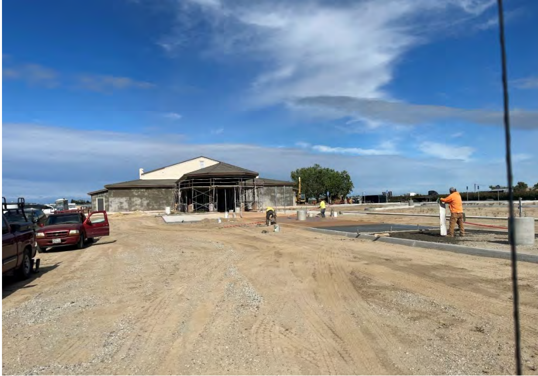
View west of Event Center under construction (east side of building).
