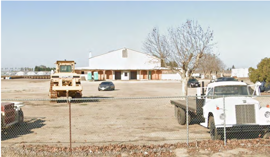
View of east side of building for N. Madera Ave.
