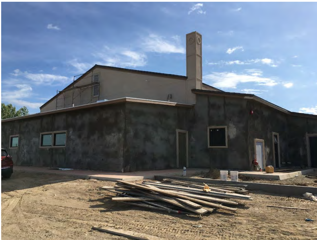
View of west side of building.
