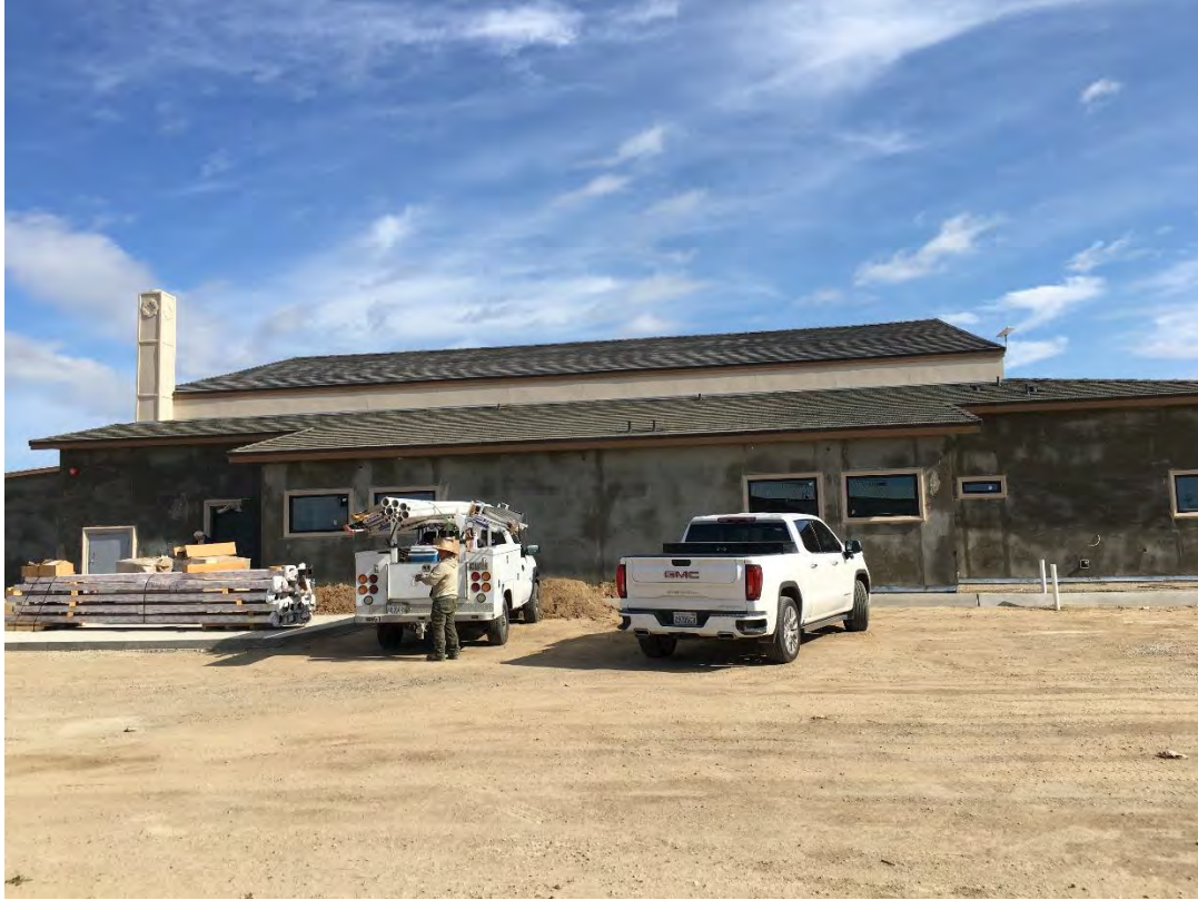
View of south side of building.
