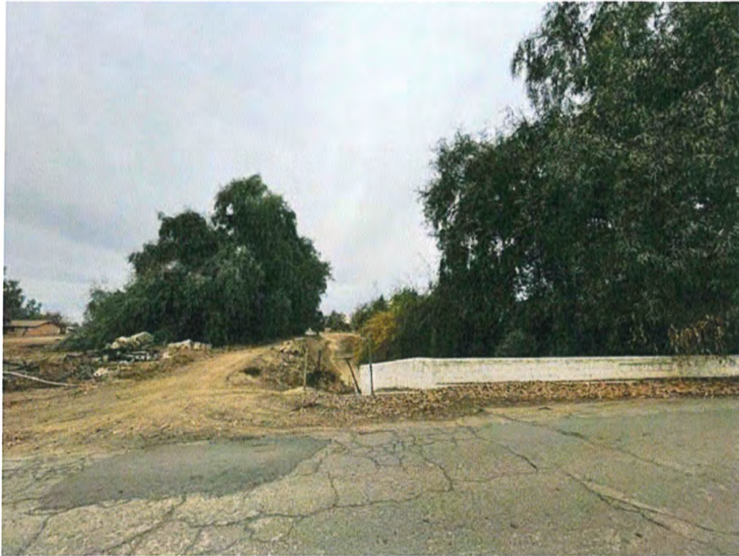
West view facing the canal.
